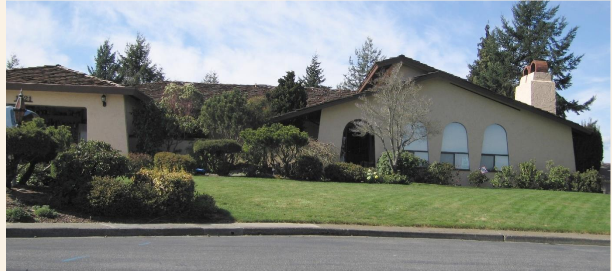
HOUSE TACOMA C.19774
