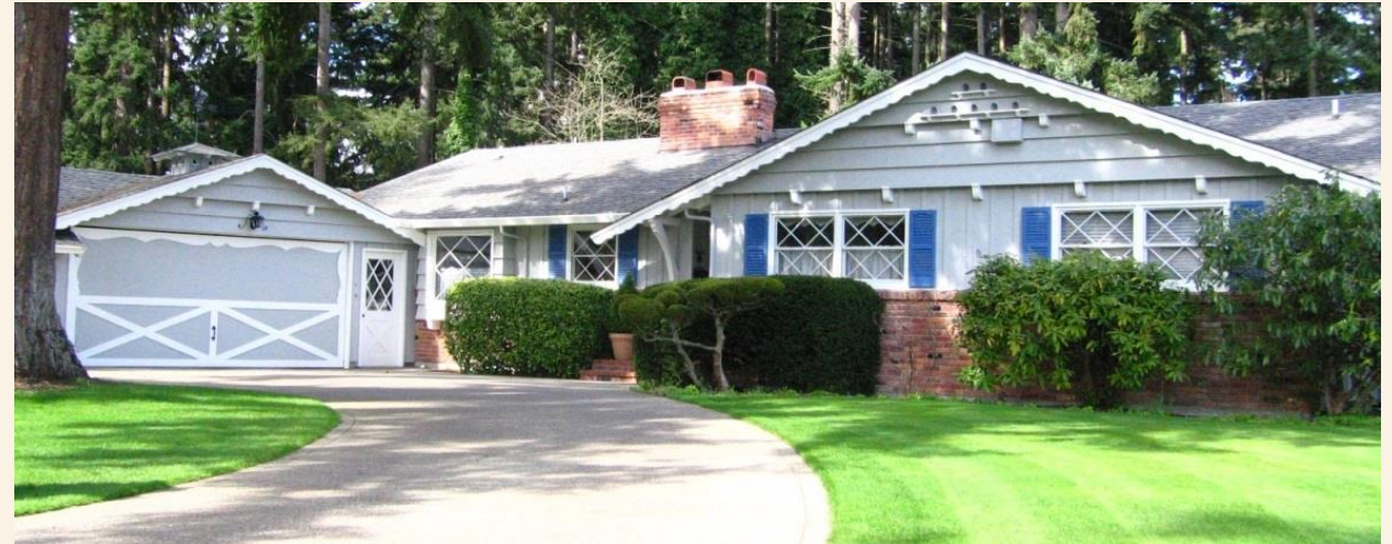
HOUSE TACOMA, C.1960
