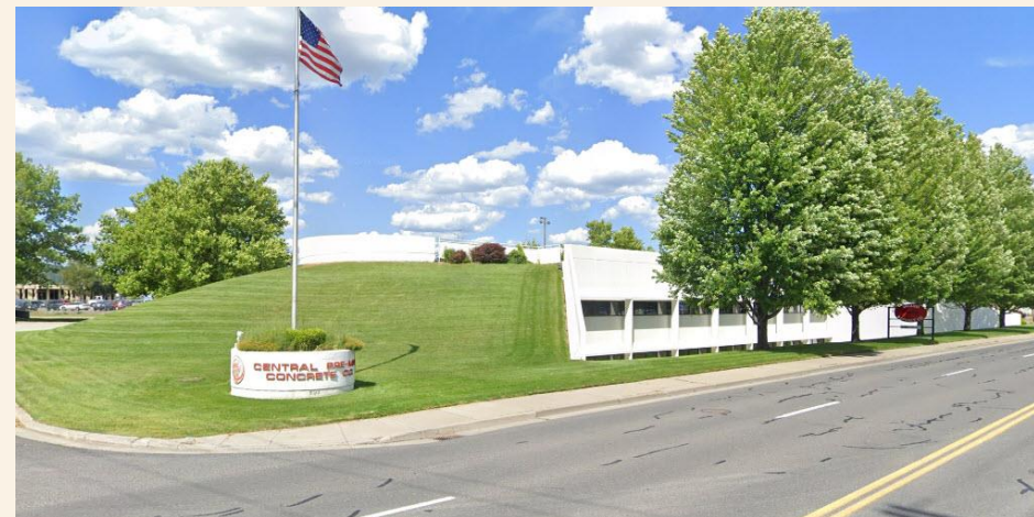
CENTRAL PREMIX CONCRETE | SPOKANE, 1980
