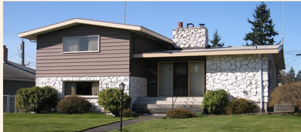
HOUSE | TACOMA, C.1968
