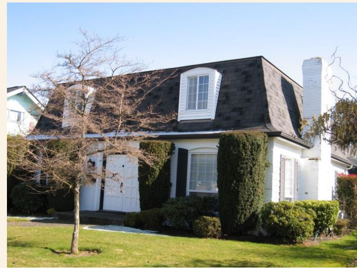
HOUSE | TACOMA, C.1980
