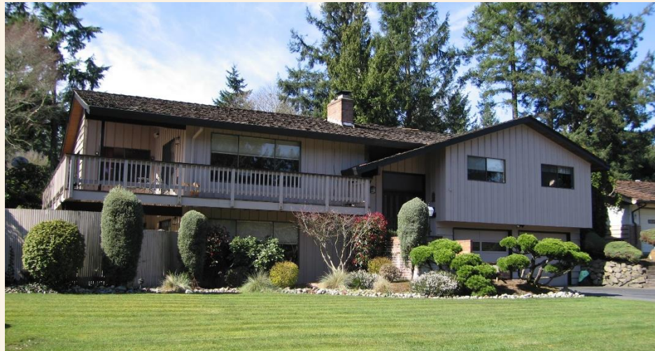
HOUSE | TACOMA, C.1968
