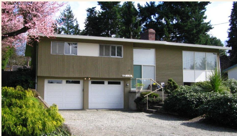
HOUSE | TACOMA, C.1970
