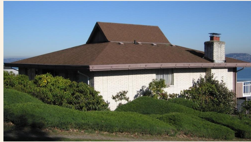
HOUSE | TACOMA, C.1975
