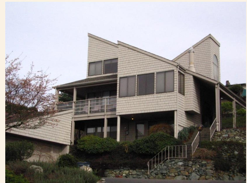
HOUSE | TACOMA, C.1978
