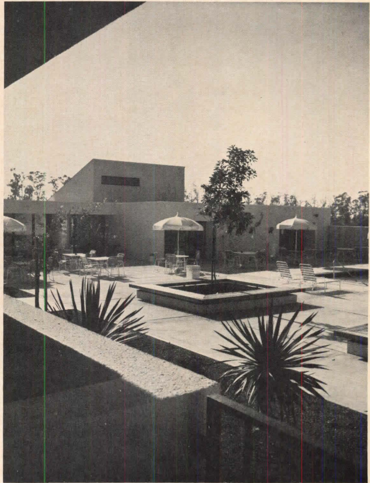
The Meadows, a 356-unit mobile home park on Irvine Ranch in California, is the design of Riley/Bissell/Associates. A main attraction is the community center and clubhouse which provides both indoor and outdoor recreation. It has such amenities as a laundry room wing, a huge kitchen, dining room and a roofed tournament shuffleboard court.
