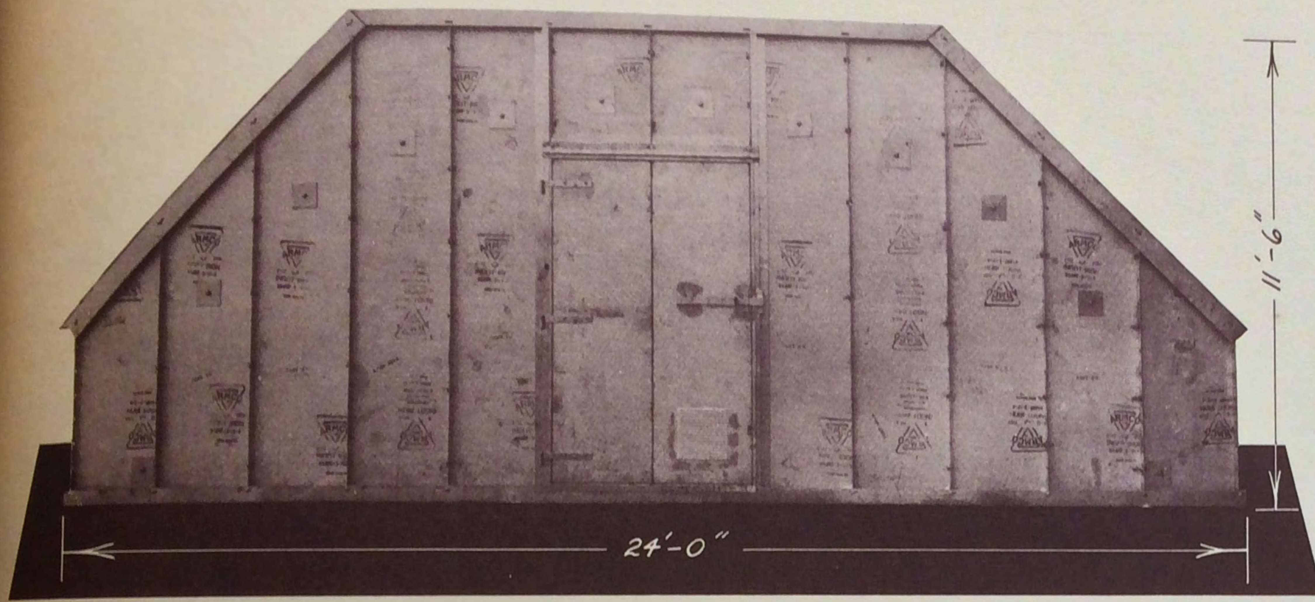
ARMCO MULTI PLATE MUNITION STORAGE MAGAZINE (FRONT VIEW)
