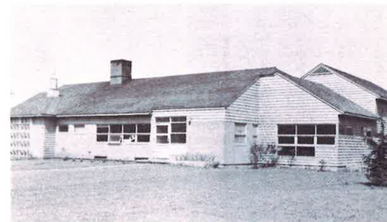
Fourth Plain Village Center now used by the City of Vancouver for its Water Department.
