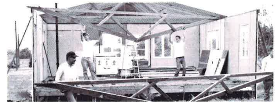
The scenes on this page were typical of postwar activity in the various housing projects. Four entire "cities" were torn down and moved away or reduced to salvage. The pictures show a McLoughlin Heights prefab being dismantled and carted off. These were re-erected throughout the Pacific Northwest on farms, in mountains, at beaches and at public works projects, like the 150 units that were used by the Bureau of Reclamation at Grand Coulee dam (in foreground of picture below).
