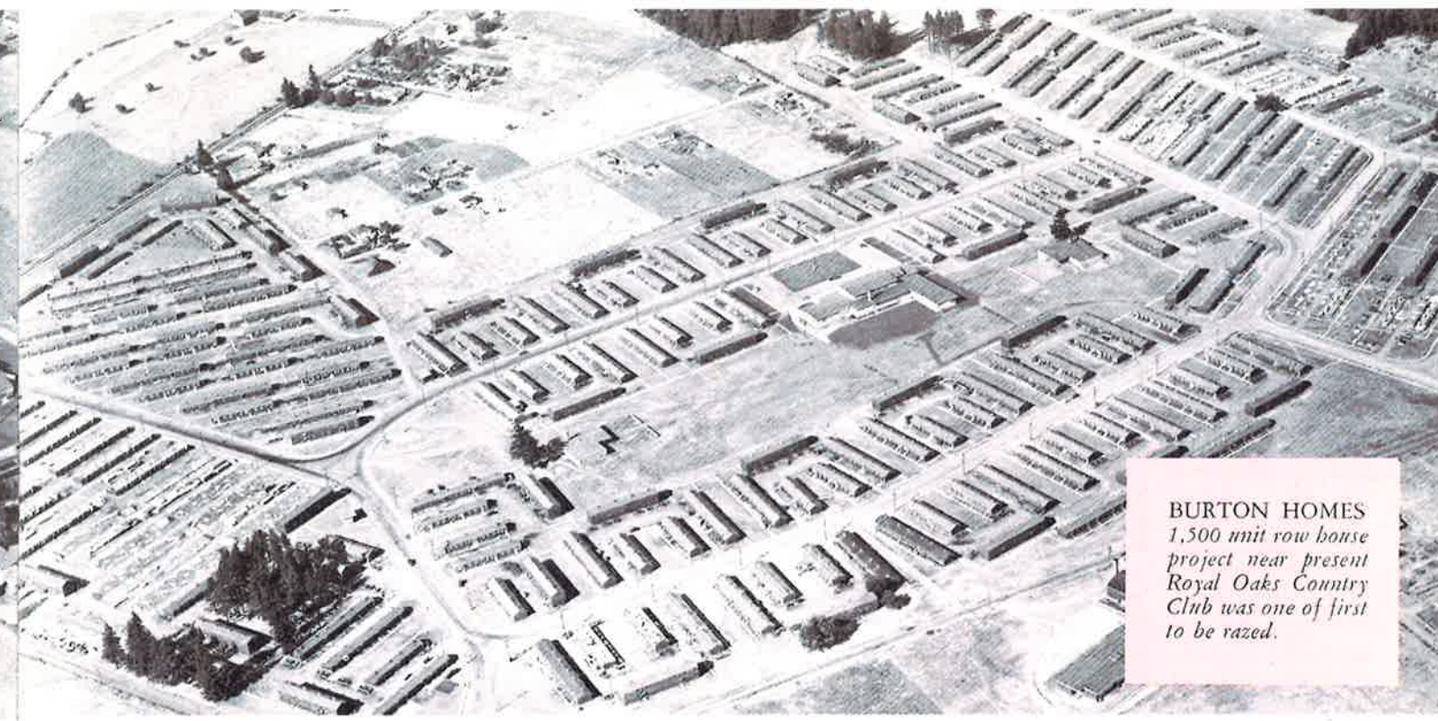
FOURTH PLAIN VILLAGE 200 unit permanent project, served Ross substation and public employees.
