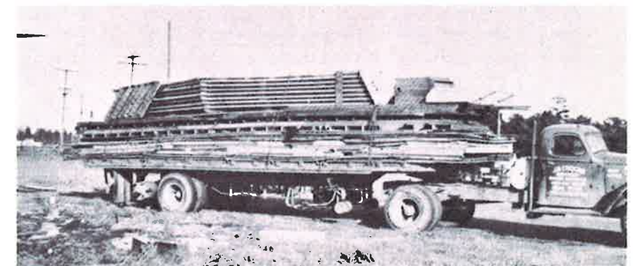
The scenes on this page were typical of postwar activity in the various housing projects. Four entire "cities" were torn down and moved away or reduced to salvage. The pictures show a McLoughlin Heights prefab being dismantled and carted off. These were re-erected throughout the Pacific Northwest on farms, in mountains, at beaches and at public works projects, like the 150 units that were used by the Bureau of Reclamation at Grand Coulee dam (in foreground of picture below).
