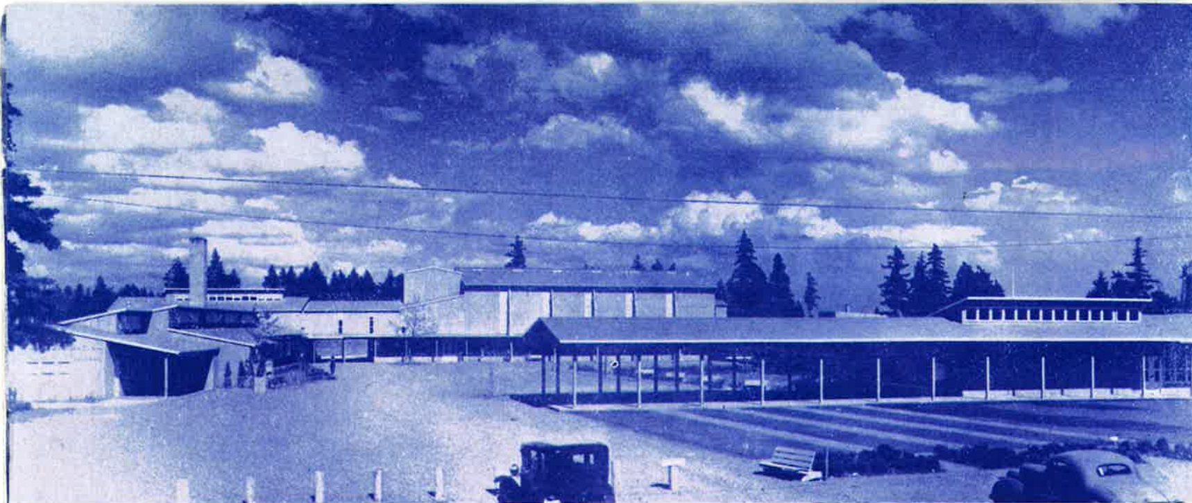
The administration-community center pictured above houses the central offices of the Housing Authority. This building has been called the finest of its kind on any U. S. war housing project.
