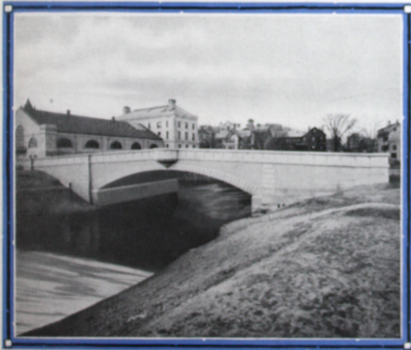
Armory Bridge, West Medford, Mass. ALPHA CEMENT used exclusively.
