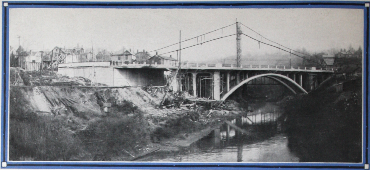
New Decker's Creek Viaduct, Morgantown, W. Va. 24,000 bags of ALPHA CEMENT used
