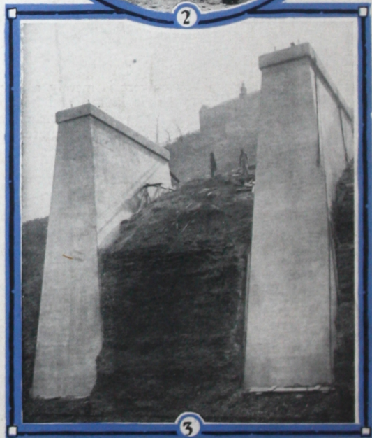
Work on Bloomfield Bridge, Pittsburgh, Pa.
