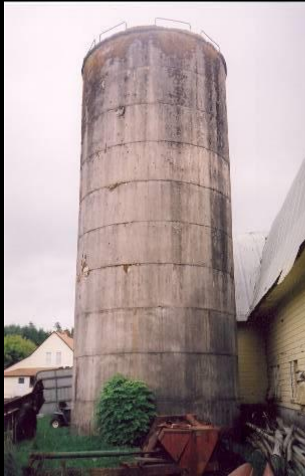
Poured Concrete Silo
