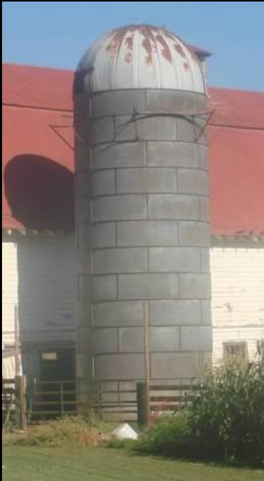
Steel Paneled Silo
