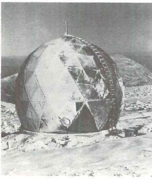
31-foot, 3,000 pound geodesic dome atop Mt. Washington, N.H., stood 200 mph winds during a year test for use on the DEW Line.
