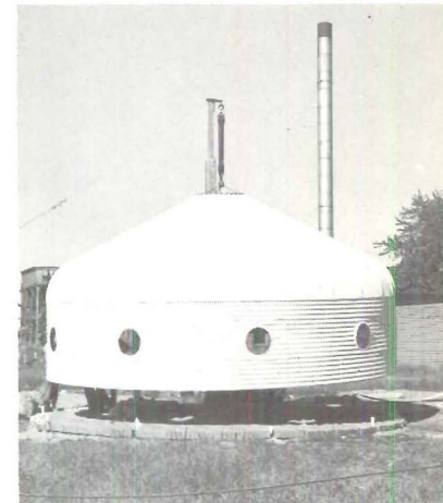
The Dymaxion Deployment Unit, 1940, a 4,000 pound grain bin of a house, was tooled for a production rate of 1,000 per day.
