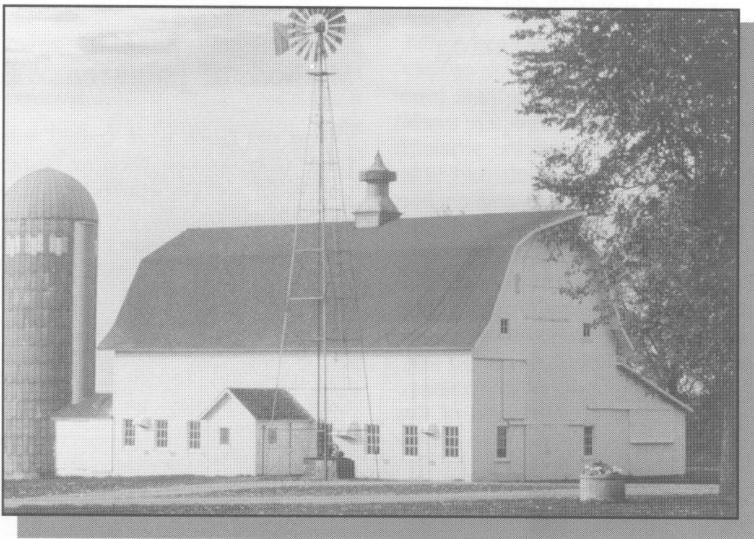
Black-painted plywood placed behind glass keeps appearance of windows, which were covered on the inside to convert this barn for farrowing hogs.
