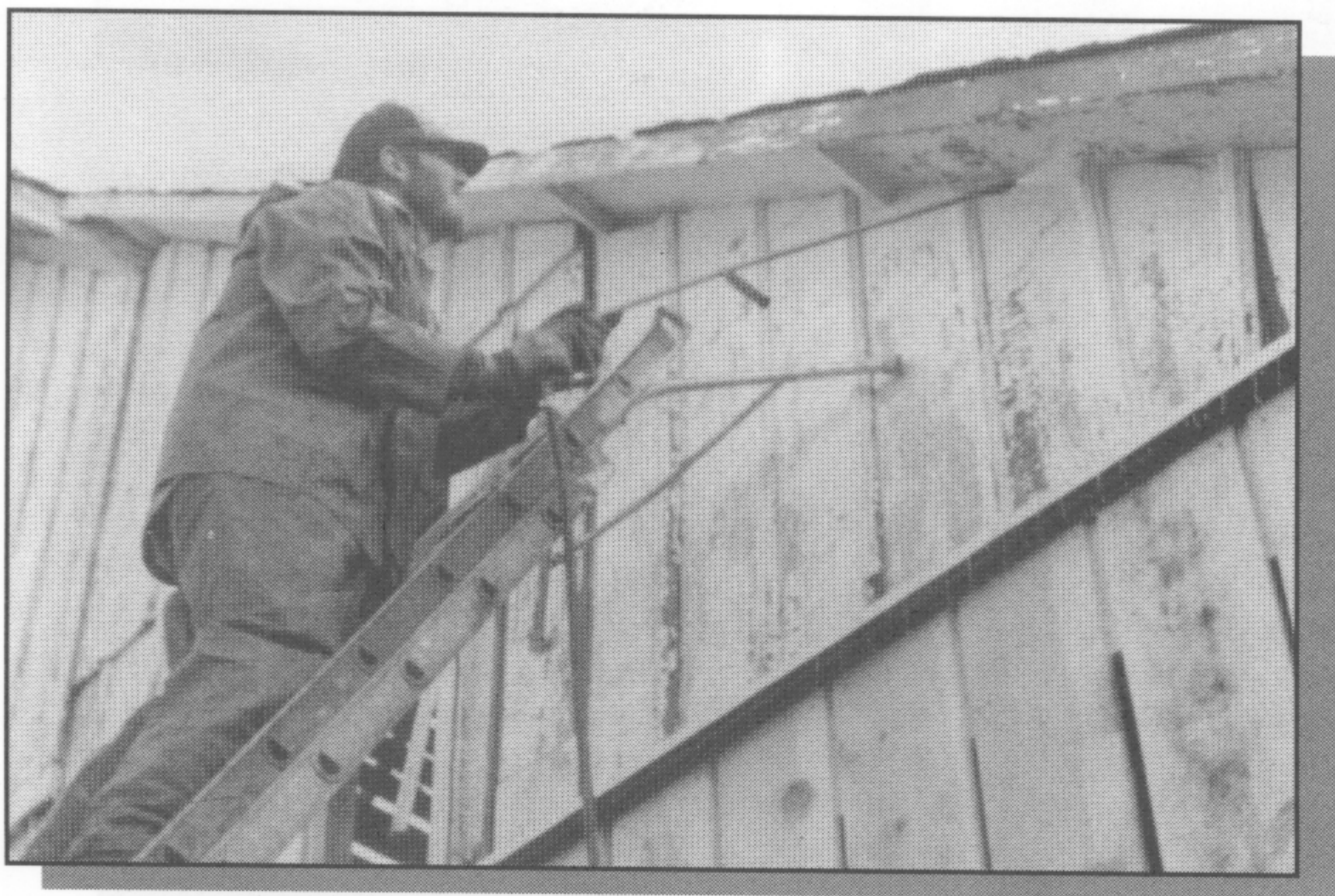
Power washing removes loose, peeling paint.
