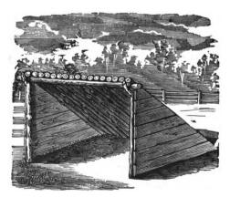
Fig. 116—SHELTER OF POLES AND BOARDS
