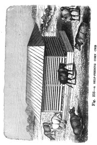
with battens over the cracks. The crib should be placed at least a foot above the ground, so that it will not harbor rats. The one shown in the engraving is supported by two large sills. Pillars of brick or blocks of wood can be used.
