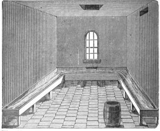
Fig. 277—Interior of spring house, with elevated trough
