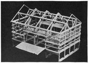
Fig. 5-MODEL OF A PLANK FRAME BARN
