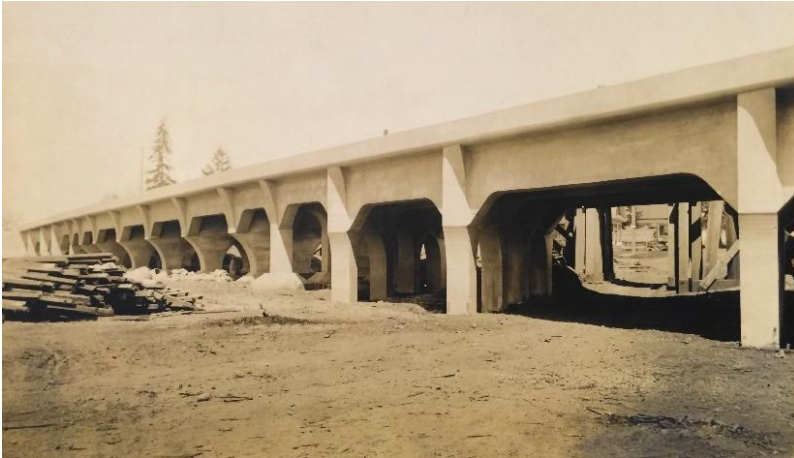
Figure 18. SP&S reinforced-concrete viaduct. Source: MHS.
