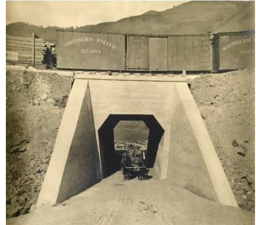
Figure 19. SP&S reinforced-concrete culvert. Source: MHS.
