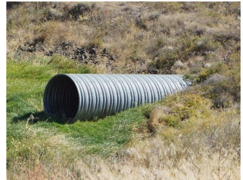
Figure 42. SP&S metal pipe culvert.
