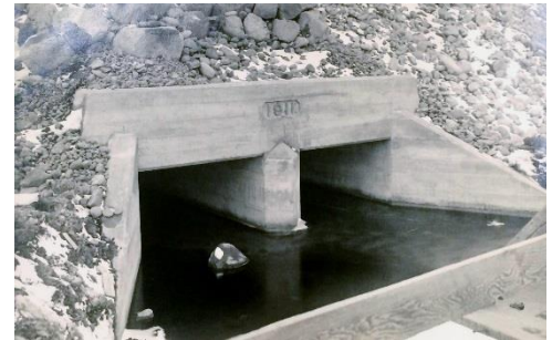
Figure 41. SP&S two-chamber concrete culvert.
