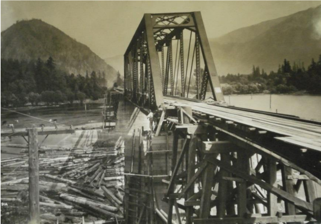
Figure 6. Close up of frame on pile trestle, Wind River Bridge, 1913. Source: Oregon Historical Society (OHS).
