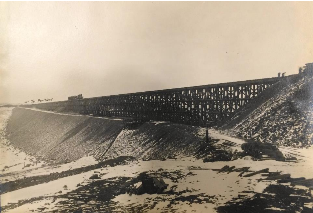
Figure 8. typical SP&S trestle, ca.1908. Unknown location. Source: Minnesota Historical Society (MHS).
