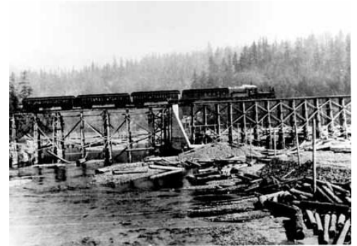
Figure 21. SP&S framed trestle at Wind River.
