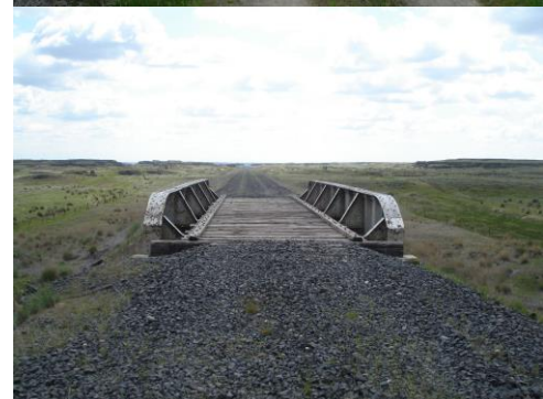
Figure 25. SP&S “through-plate” girder span, Paxton Bridge.
