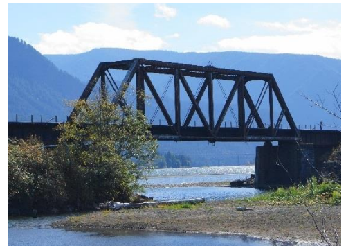
Figure 29. SP&S Pratt truss bridge near Stevenson, WA.
