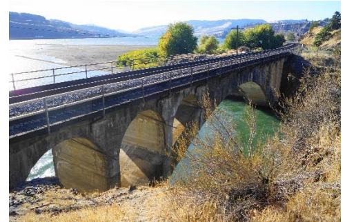
Figure 33. SP&S reinforced-concrete arch bridge over Klickitat River.
