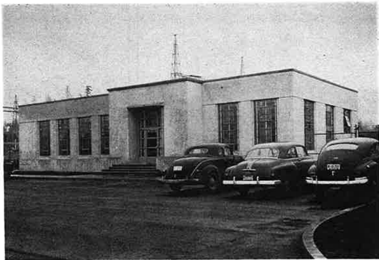
CONTROL HOUSE Bonneville Power Administration Tomwater, Washington
