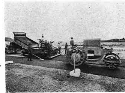
Paving Drive-In Theatre
