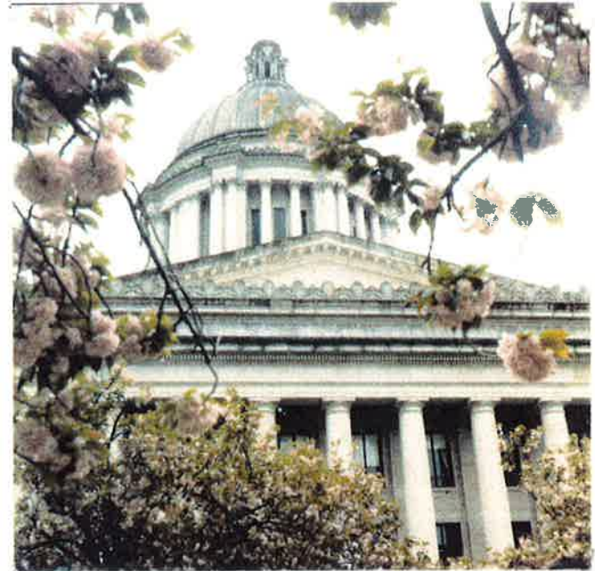
Legislative Building Stonework Repair
