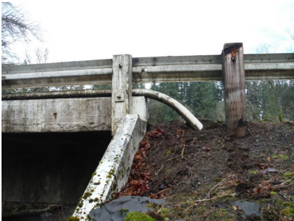
Utility pipe and guardrail along southern side of Bridge 65 2015
