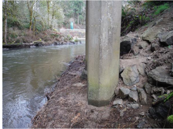
Concrete pilings on east shore of Cedar Creek 2015
