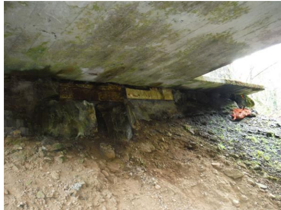
Eastern abutment, Bridge 65 2015
