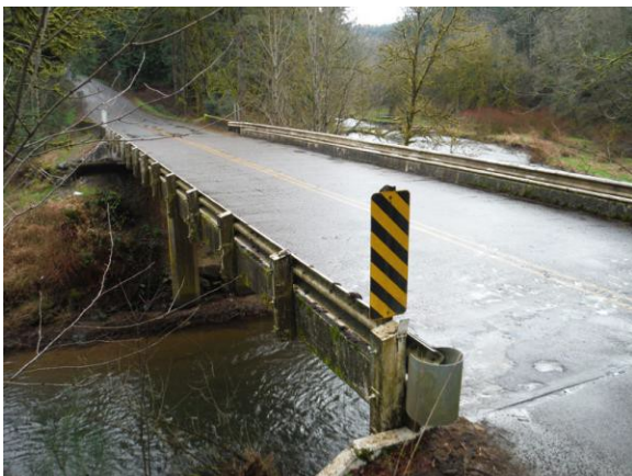
Utility pipe and guardrail along southern side of Bridge 65 2015
