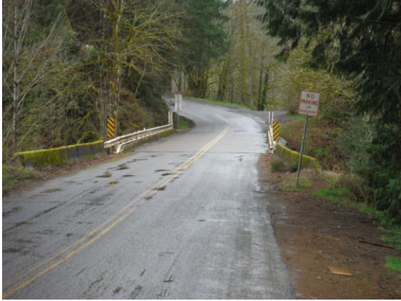
Bridge 65, looking west 2015
