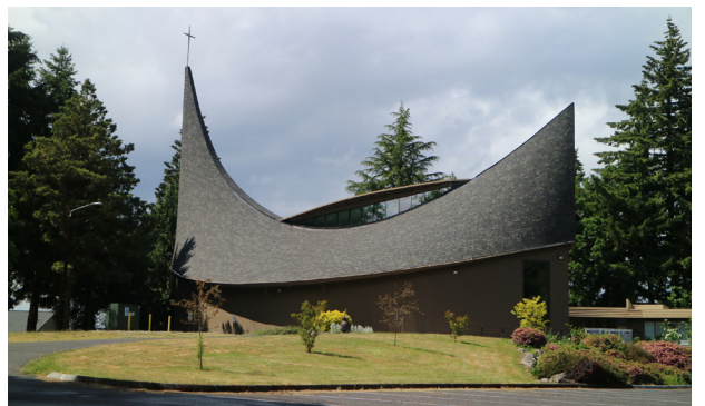
Above: Split Level form at 3414 NE Royal Oaks Dr., Vancouver ; A-Frame form at 5700 SE Riverdale Way, Vancouver; Sawtooth Roof/Folded Plate form at 507 E Main St., Battle Ground; Hyperbolic Paraboloid form at 1220 NE 68th St., Vancouver
