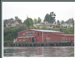
SEBASTIAN STUART COMPANY Built in 1915, the now vacant Sebastian Stuart Company building originally served as a salmon cannery. In 1937, tuna canning operations were added in the facility, establishing the first tuna cannery in the Puget Sound.
