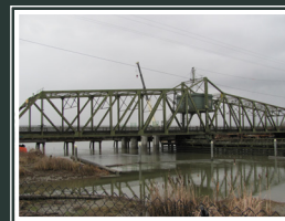
SNOHOMISH RIVER BRIDGE This ca. 1920s steel truss pivot bridge was designed to rotate on its midpoint, highlighted by the
