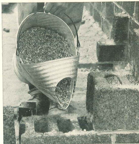
Increased insulation of concrete masonry walls may be provided by filling cores in the units with a granular insulating material.
