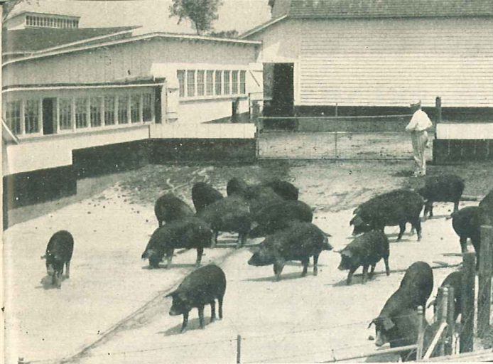
The hog feeding floor is sometimes built with a slope of \frac{1}{4} in. per foot so that it will clean by flushing with water from a hose.
