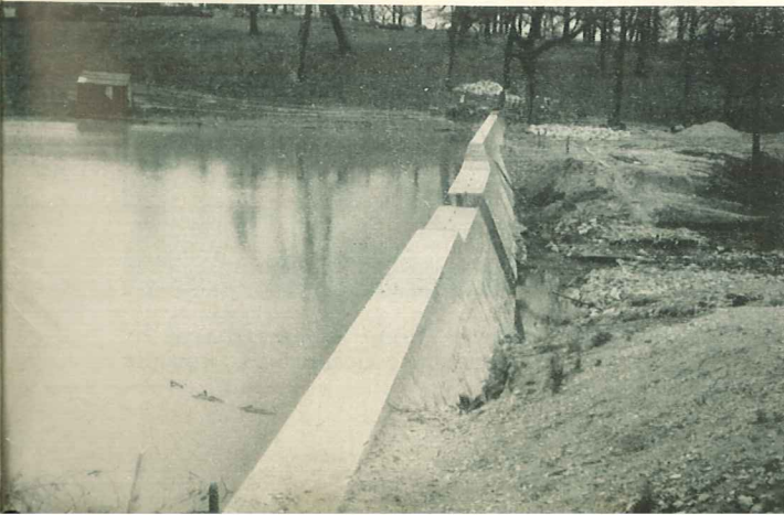
This cast-in-place concrete dam has permanently stopped destructive gullyng and created a farm pond valuable for stock water supply.
