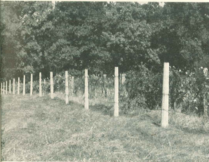
These concrete posts, erected in 1914 on the Iowa Experiment Station Farm at Ames, were 25 years old when this photograph was taken. They will continue to give trouble-free service for many more years.
