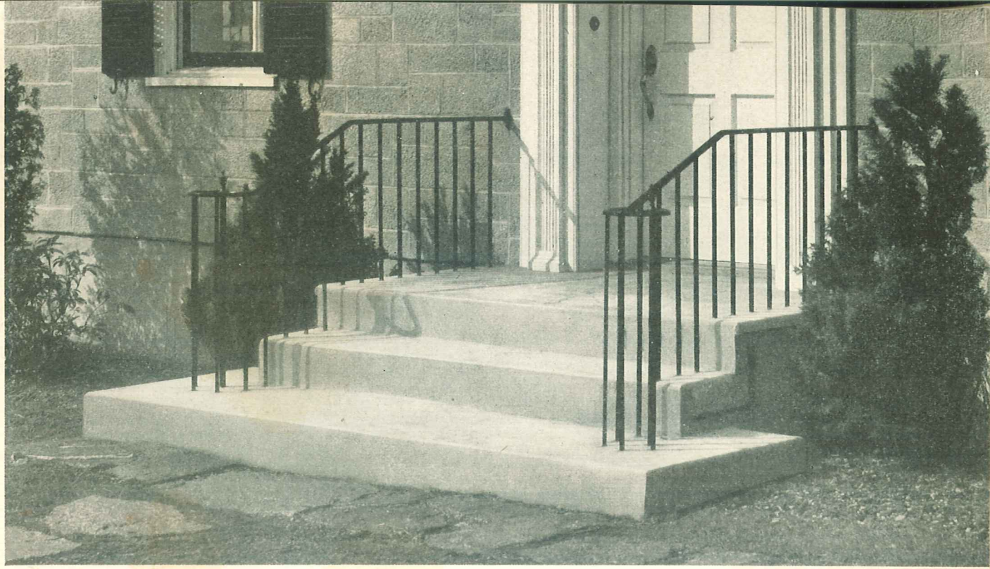
Well built concrete steps help provide an attractive entrance for the home.
