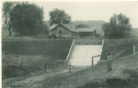
Shallow reinforced concrete spillway or flume for an earth dam which is filling in and leveling a barnyard that was becoming seriously eroded.
