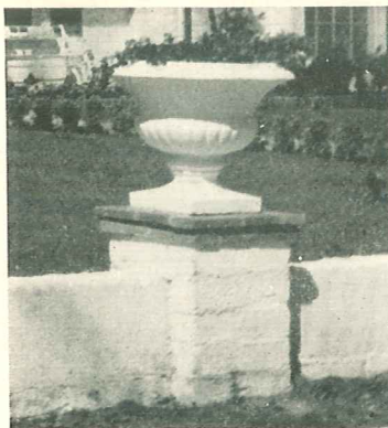
This concrete flower urn is mounted on a pedestal or standard of concrete masonry and set into a low wall, thus helping to set off the yard to advantage.
