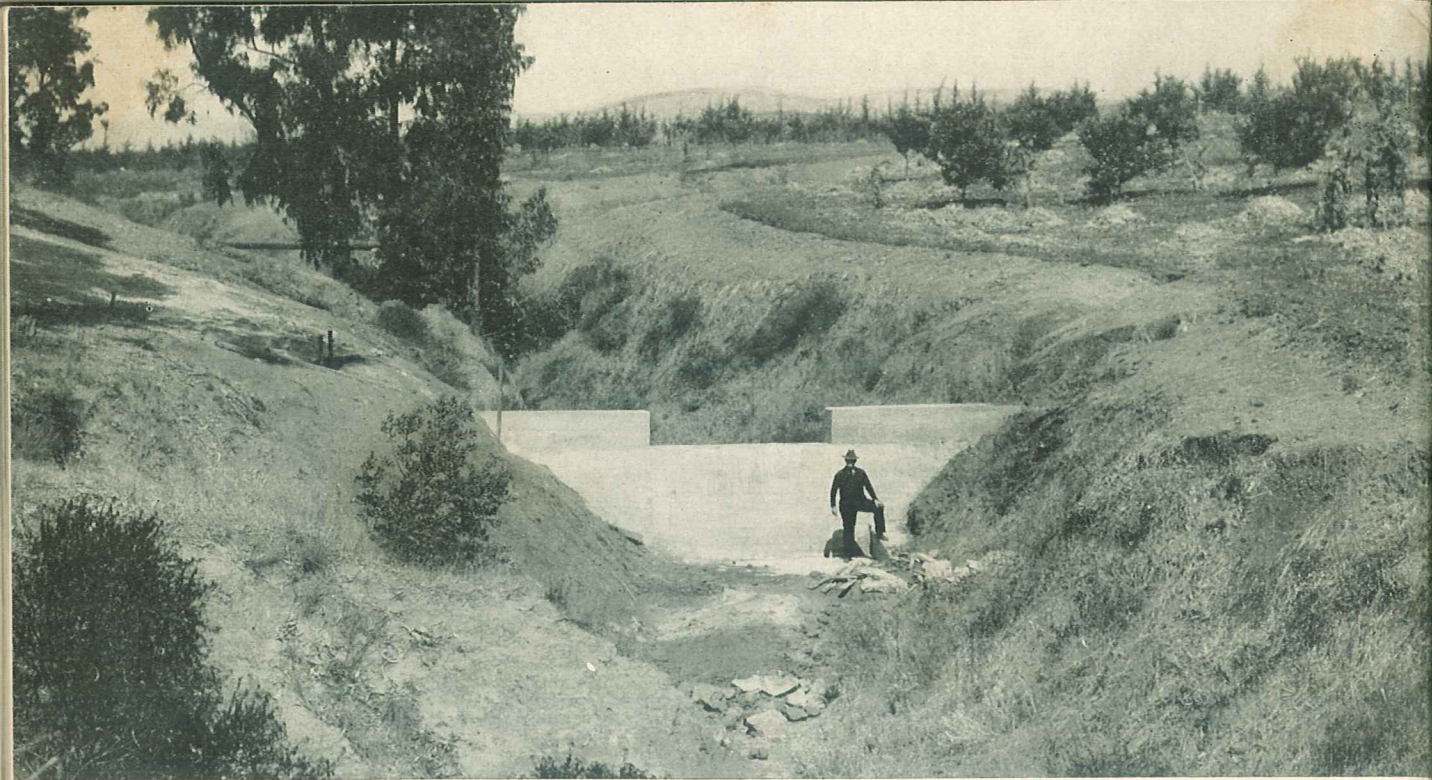
Reinforced concrete check dams stop gullying action and gradually fill in drainageways above the dams.
