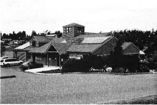
Good Example of compatible installation, below ridgeline, of photovoltaic panels on Coupeville Public Library.
