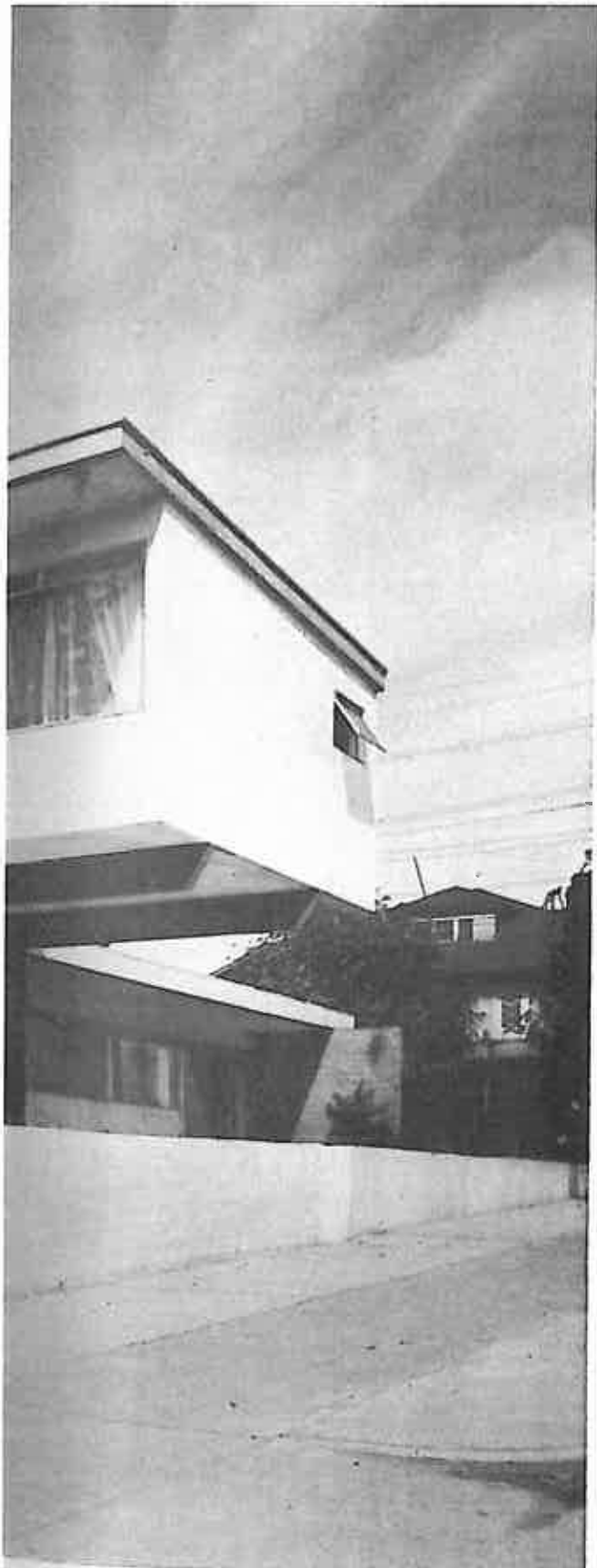
second-floor residence lies crosswise over clinic; photo: Dearborn-Massar
