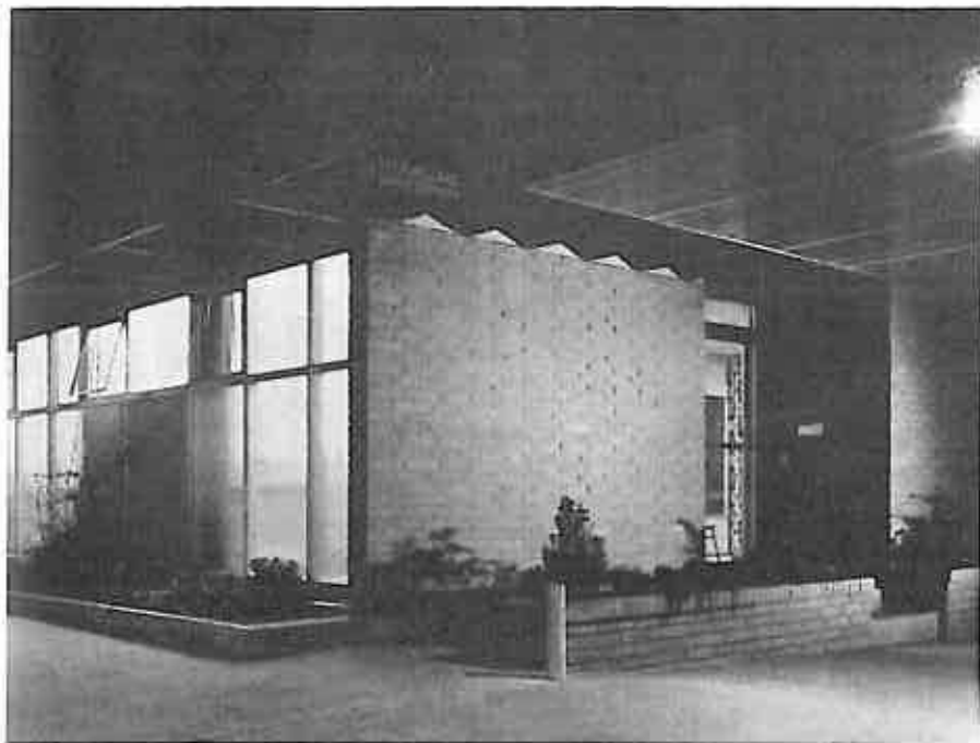
site and floor plan (left); night view of northeast corner; photo: Art Hupy
