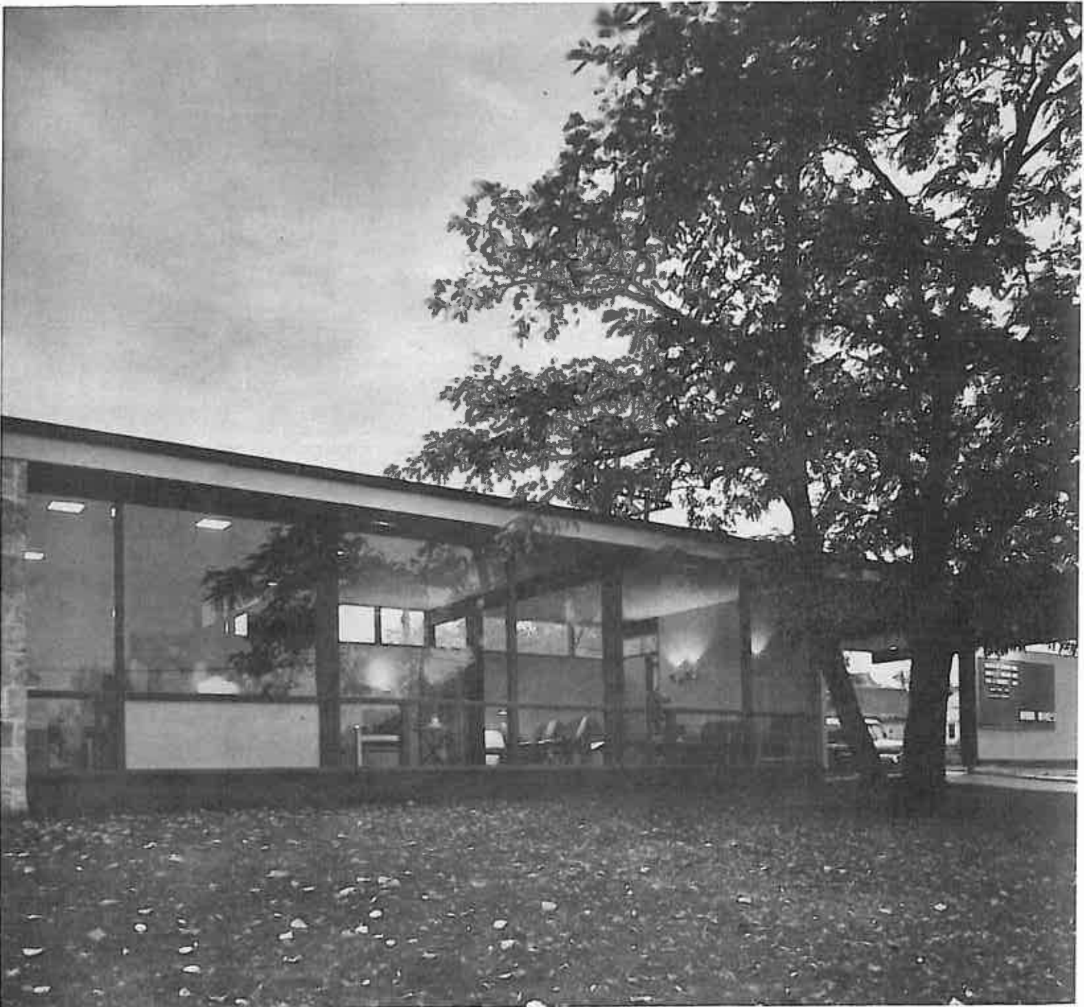
front view, looking into reception and waiting rooms; photo: Dearborn-Massar
