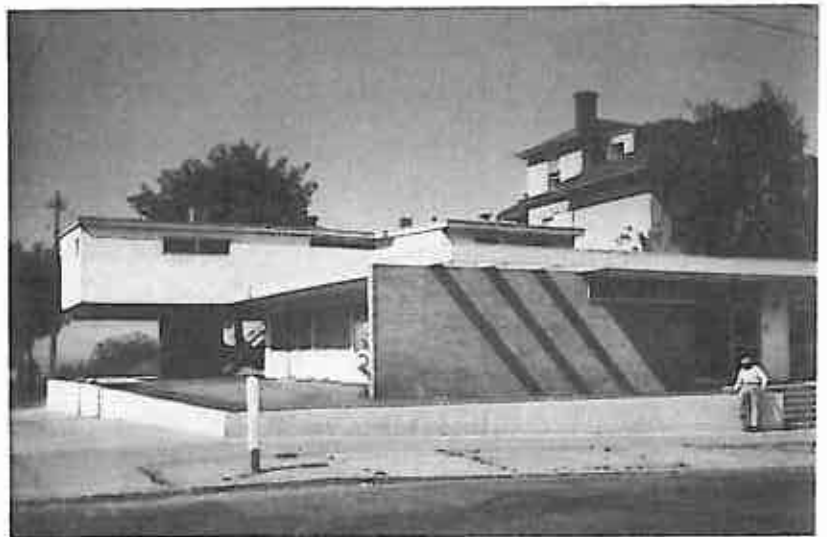
east view of exterior, showing entrance to clinic; all photos: Dearborn-Massar
