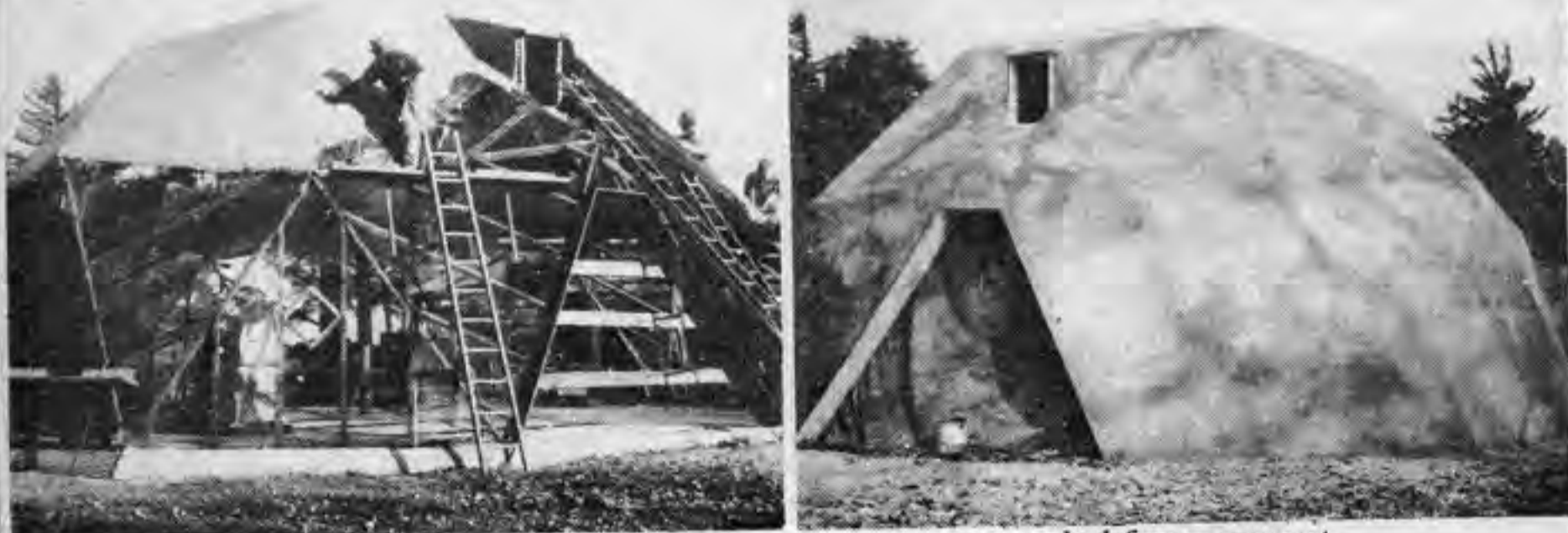
unsealed ferro cement
