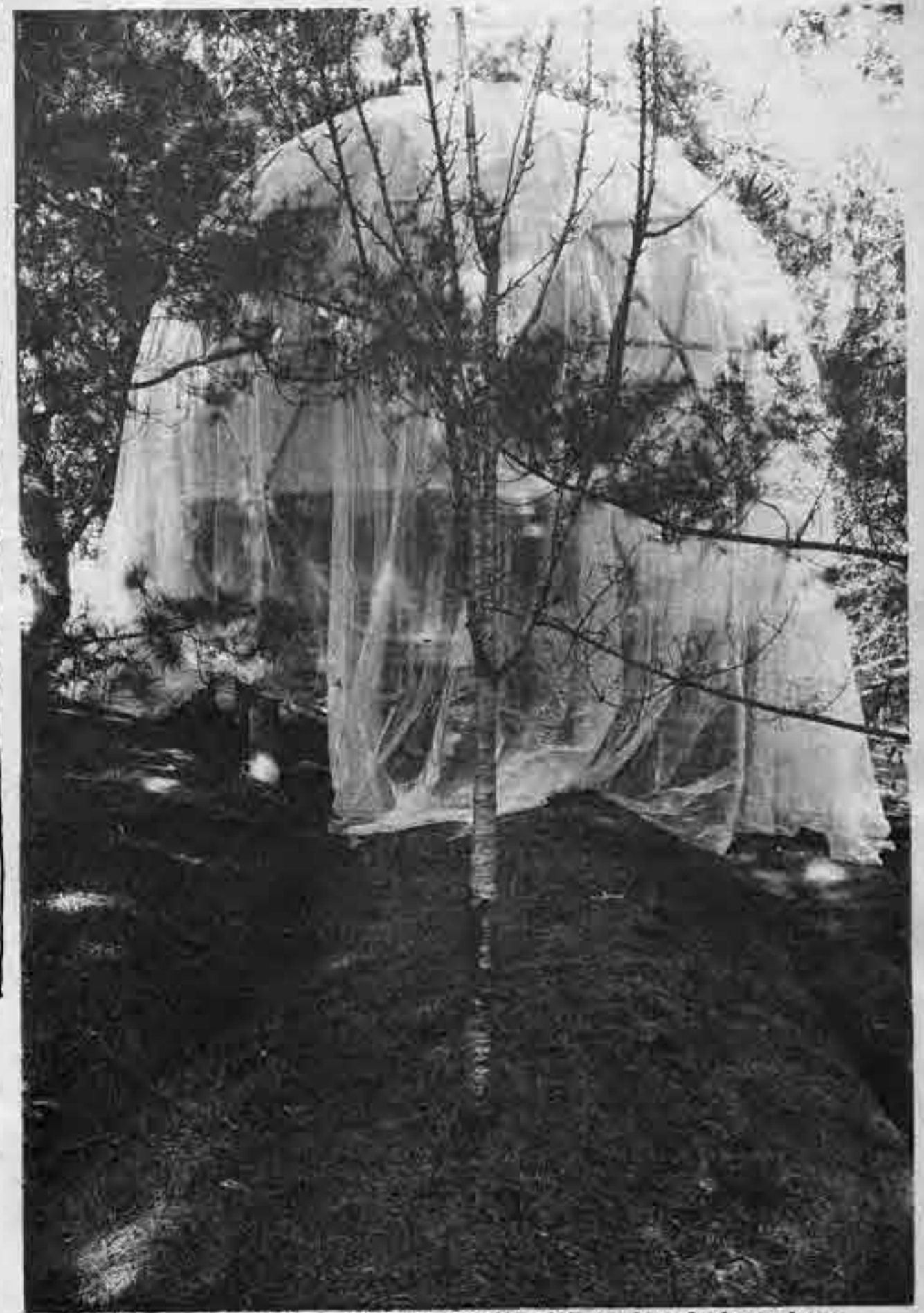
3/4 Dome temporarily covered with polyethelene bag
