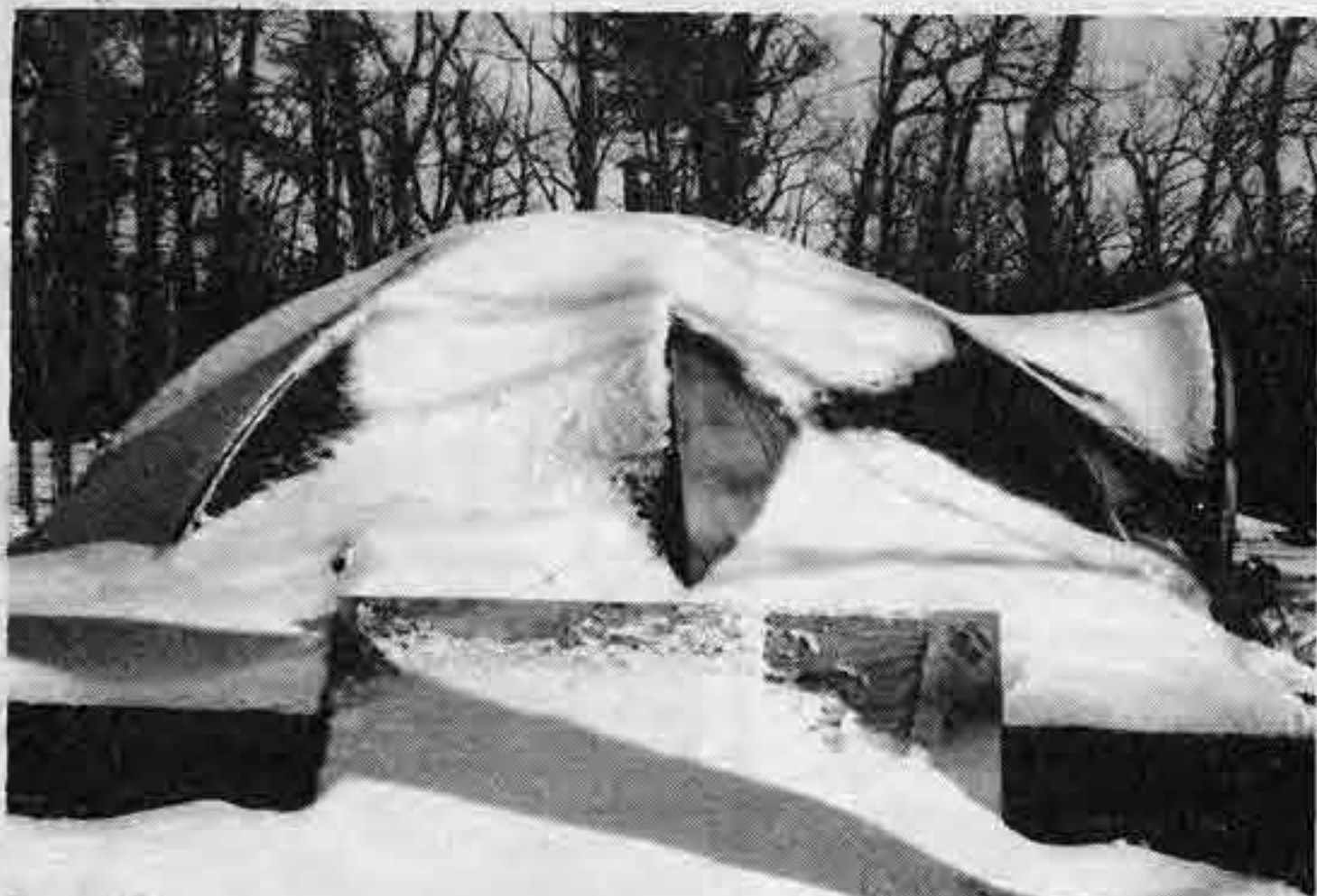
At the top the ribs were bolted to a plywood ring. The hole in the center is for chimney or summer vent.
