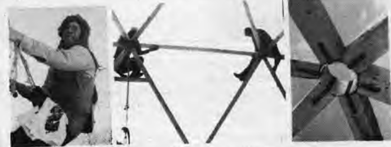
One of the advantages of a hemisphere with an even number of frequencies is that the bottom row of hubs sits flat on the floor. We strapped them to the floorboards and started going up. As we got higher we were happy to find out that the strap held all the struts in place and we never had to use support poles. We double strapped in many places just to be sure.
