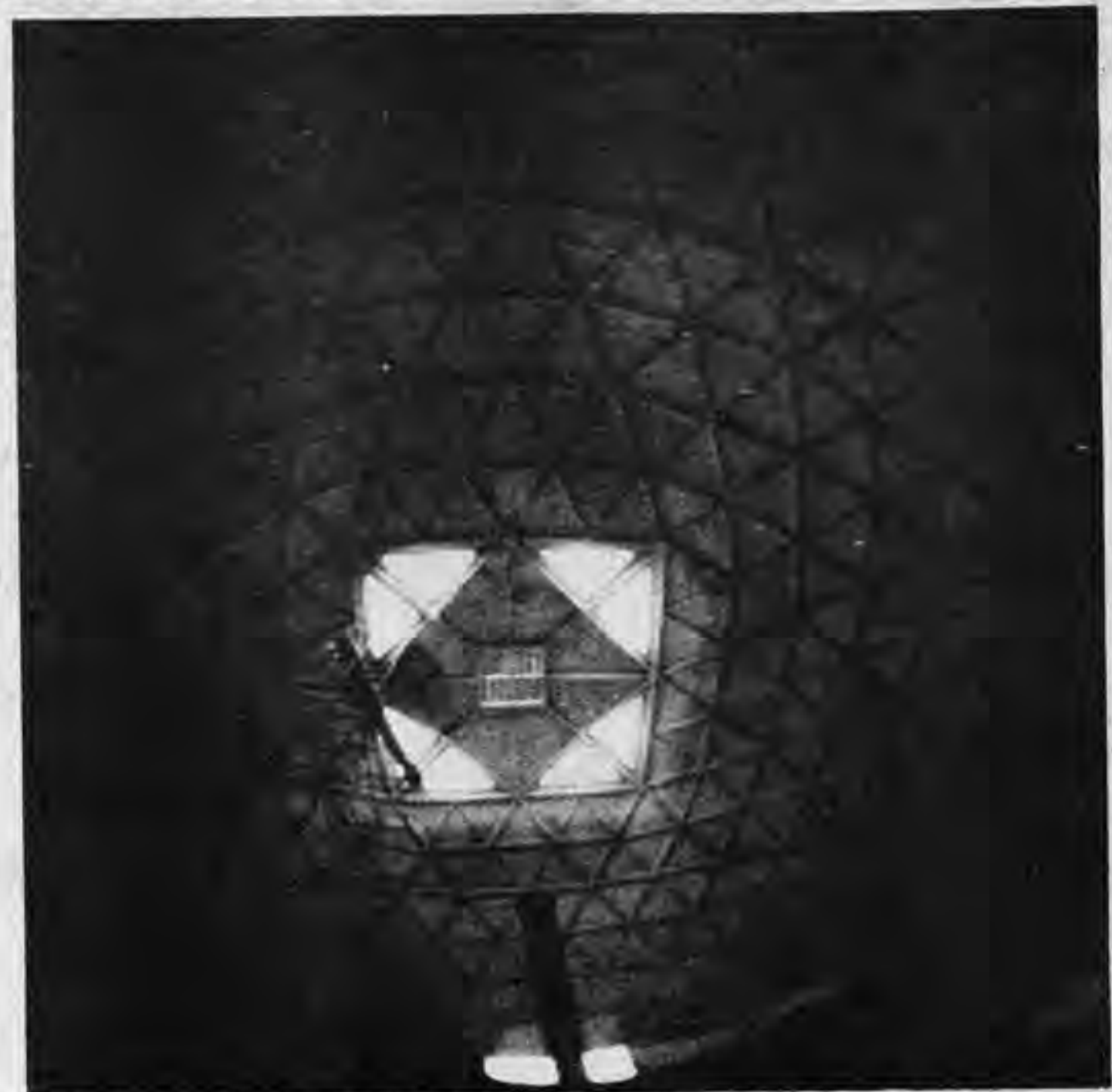
Dyna Domes produces plywood domes—2 X 4 struts, plywood skin, fiberglassed exterior, and foam-shot interior.
