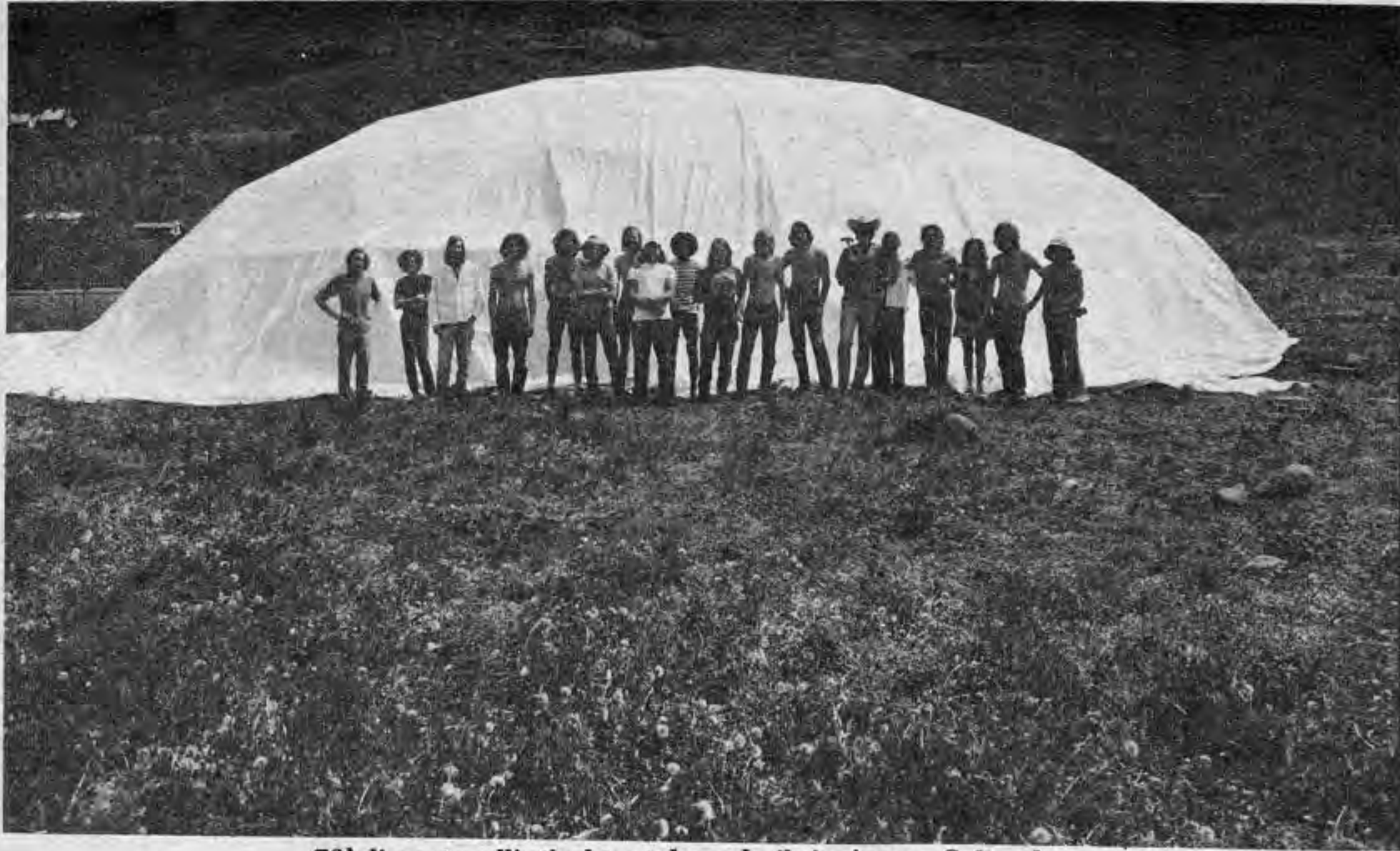
70' diameter elliptical tent dome built in Aspen, Colorado.
