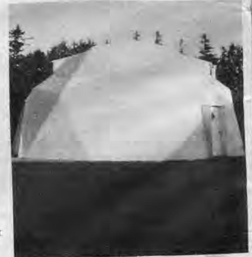
finished dome with white sealer
