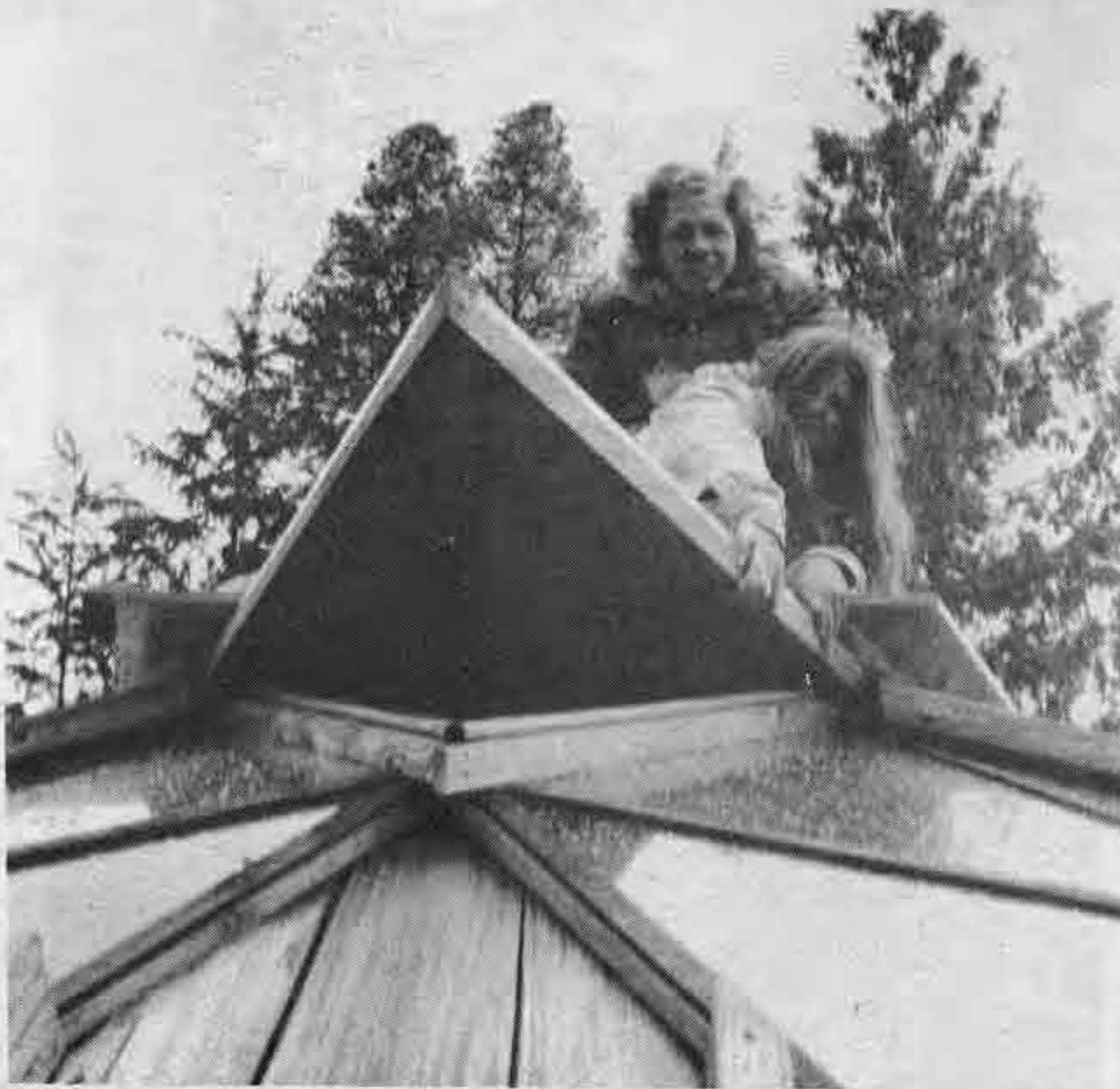
Frame is 2 X 4 members bolted to 3/4" ply gusset plates. Bolts were 1/2 usual price through a salvage yard. Works fine with dry wood; friction prevents pivoting. Green wood shrinks and requires retightening bolts.
