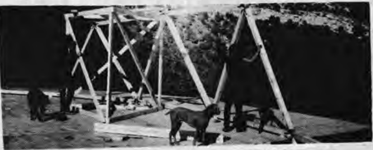
We had only built one dome before—a 22' 3-frequency Celotex covered structure which served as our kitchen while we were living in shacks and tipis—and we didn't feel ready to handle a high frequency dome. A 4-frequency hemisphere seemed to offer the best combination of simplicity and strength. Steve Baer told us it would probably work. Calculating the strut lengths from Domebook One, we built a model. We decided to use steel strap to put the dome together, and to use 4 X 4" struts and 7" diameter steel pipe hubs.
