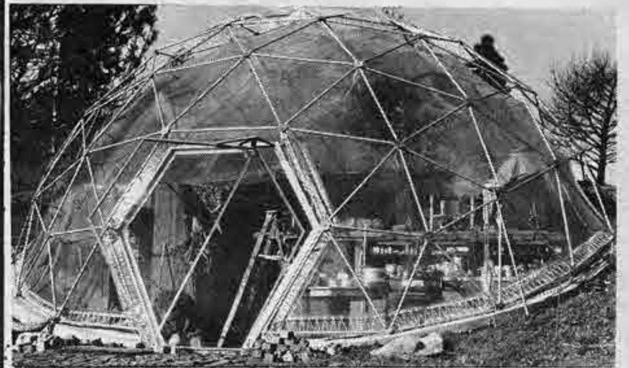
Neill Smith's door: Lexan in aluminum frame
