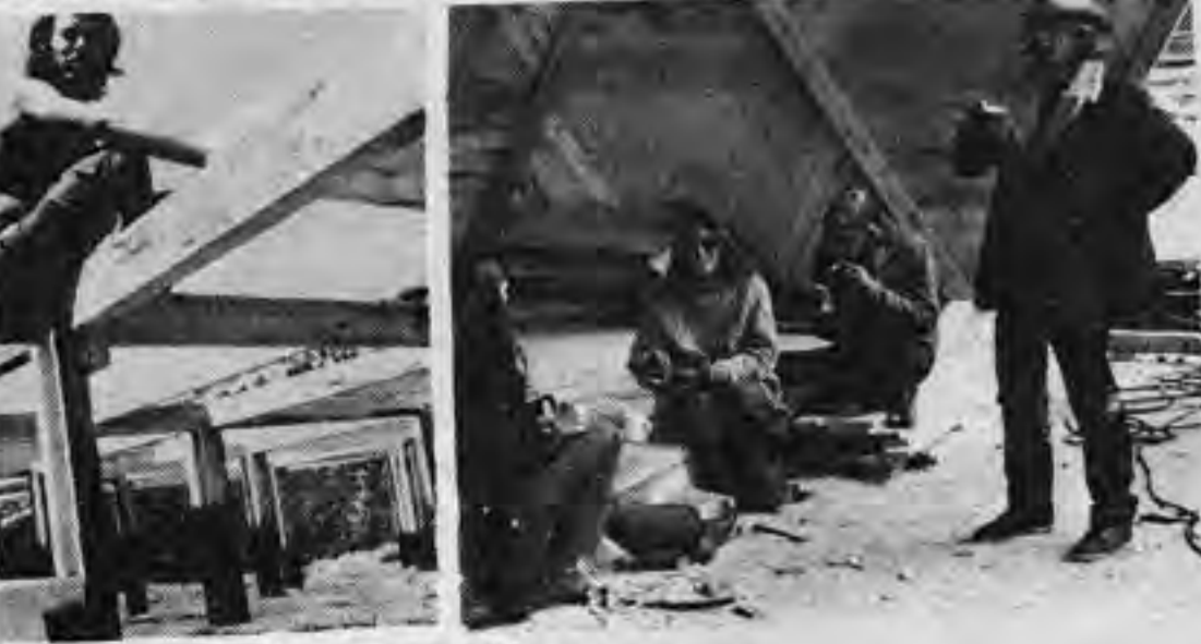
We stapled tarpaper over the joists and stringers and then laid 2 X 6" floorboards, alternating the direction of each 7 to 8 ft section so that the floor looks like a checkerboard. The tarpaper is to prevent drafts. Unfortunately, water collected between it and the boards while the floor was uncovered. It's probably still there.
