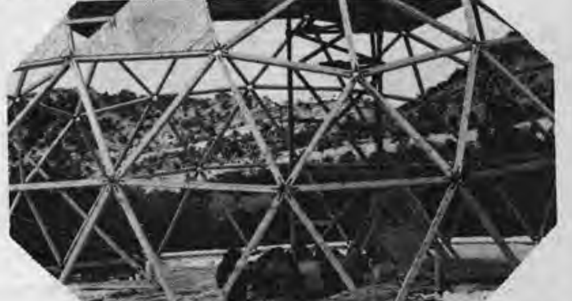
We've been living in the dome since Thanksgiving, when we finished skinning it. It's heated with two Ashley woodstoves with 20' stovepipes inside. Doors are no problem on a dome this size since they can be fit into single triangles. We haven't started on the sleeping platform yet, but eventually we'll have this 30 ft high space divided into 2 or even 3 levels. Right now we're insulating with 12 ft styrofoam 1 X 4"s—industrial waste donated by a groovy businessman. We're gluing these strips together and cutting them with a hot wire into triangular units to be painted and put up. We plan to leave the struts exposed.
