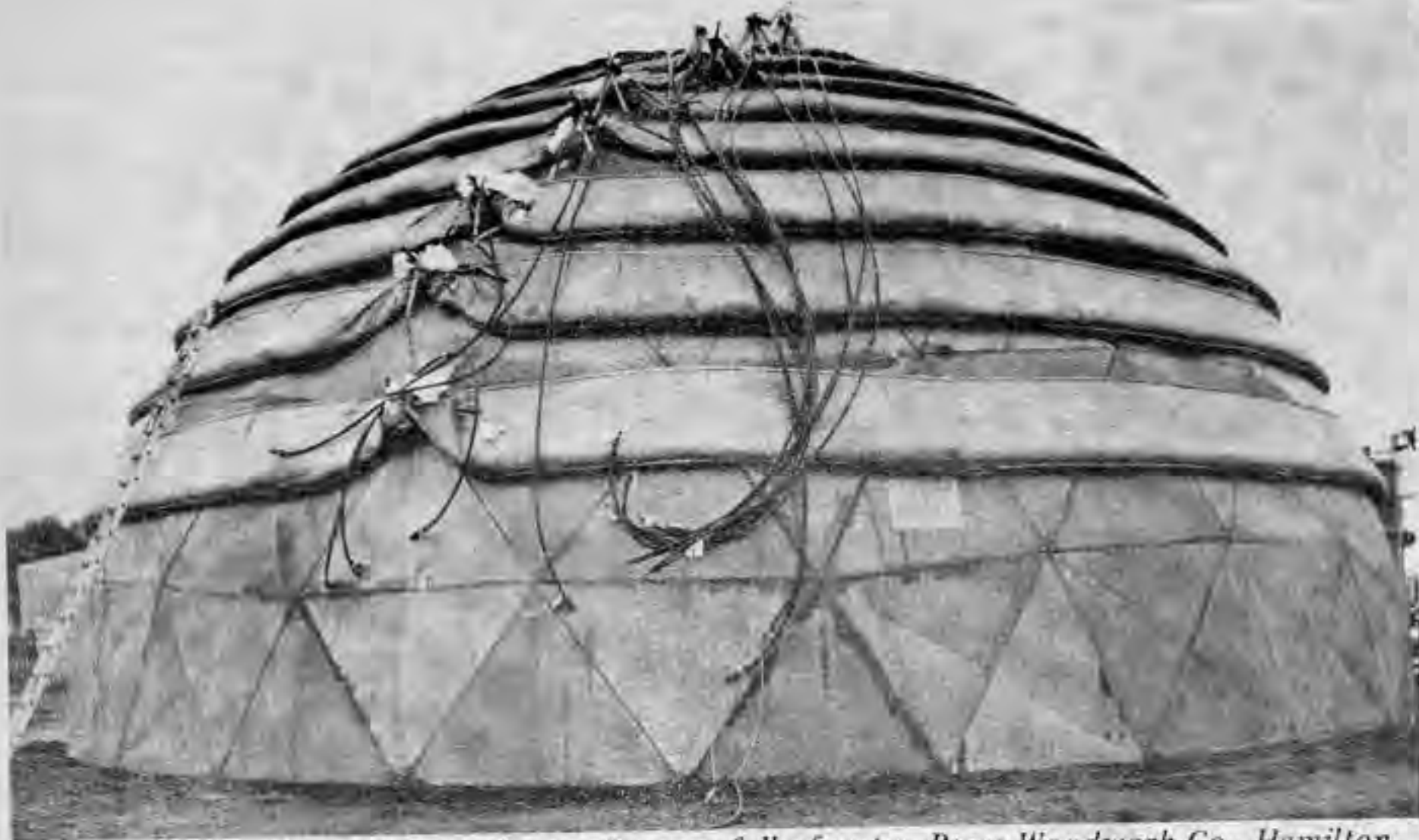
Test on plywood Pease domes. Bags are full of water. Pease Woodwork Co., Hamilton, Ohio has some valuable test data, certified by H.C. Nutting Co., testing engineers, of Cincinnati, Ohio. Dyna Domes, of Phoenix, has also made extensive structural tests.
