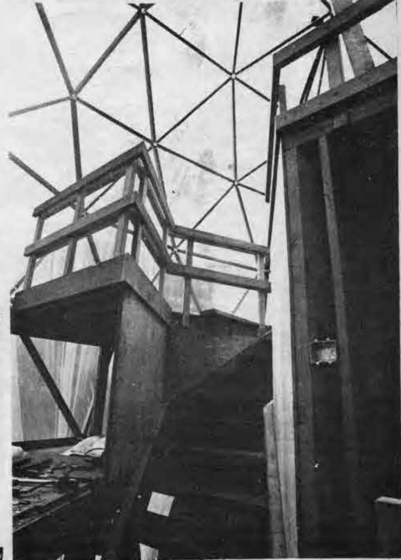
3/4 Dome temporarily covered with polyethelene bag
