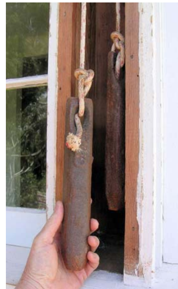
Figure 2-2. Counterweights common to many historic window systems
