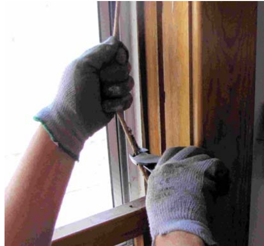
Figure 3-5. Repairing rope system
