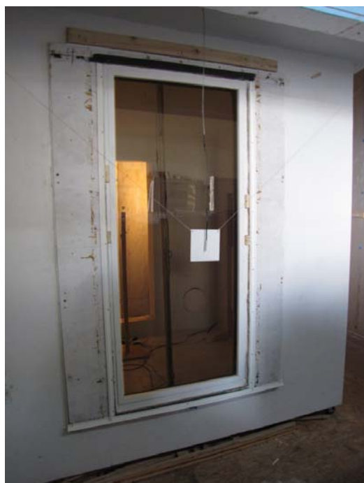
Figure 3-10. View of window with dark film installed from outside the chamber.
