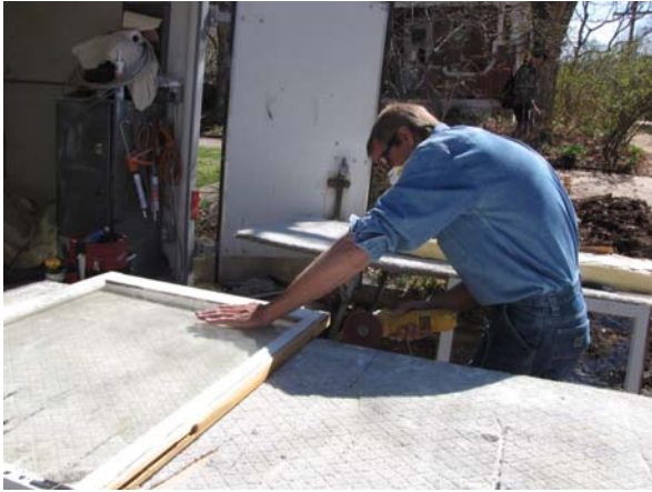
Figure 3-4. Sanding the window
