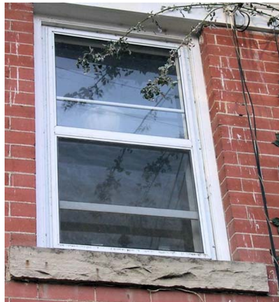
Figure 2-5. Sample window on south elevation
