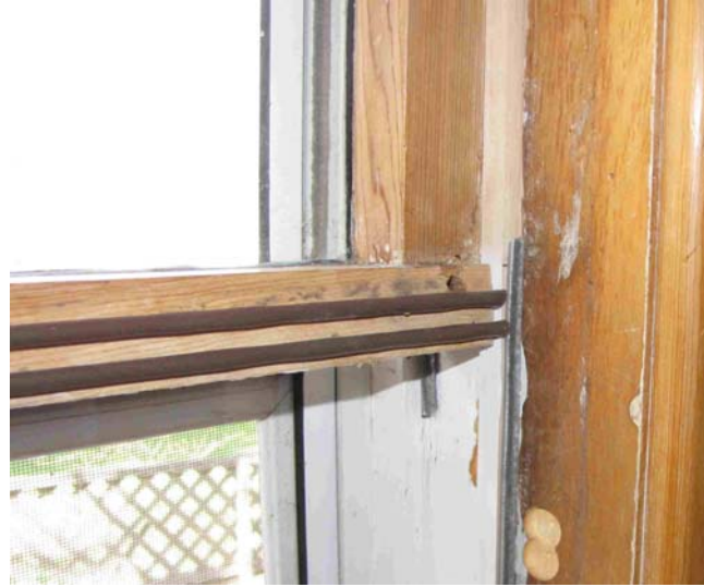
Figure 3-7. Retrofit of parting rail with weather strip
