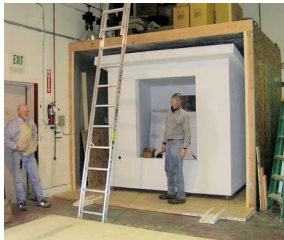
Figure 2-9. Completed test cell; outer chamber work nearing completion
