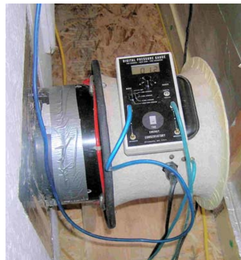
Figure 2-12. Duct blaster with manometer
