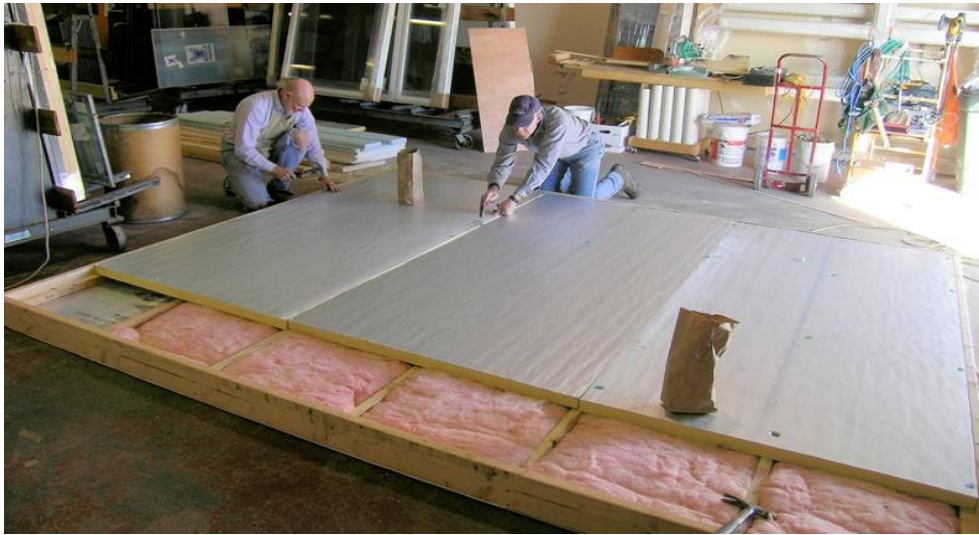
The technical team constructed a 380 pound door (see photo at left), insulated with both fiberglass and polyisocyanurate to R-25. The photos below show a winch and pulley system, suspended from steel roof rafters, used to open and close the chamber door.
