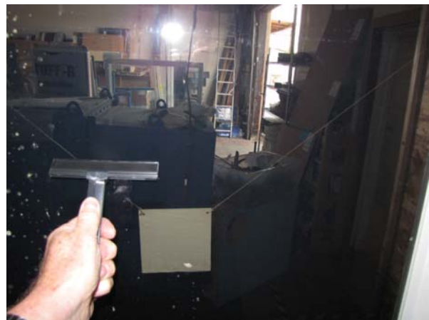
Figure 3-9. Energy Film installation
