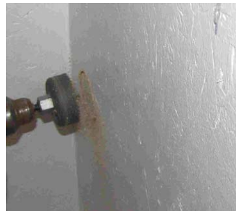
Figure 2-14. Drilling second calibration hole
