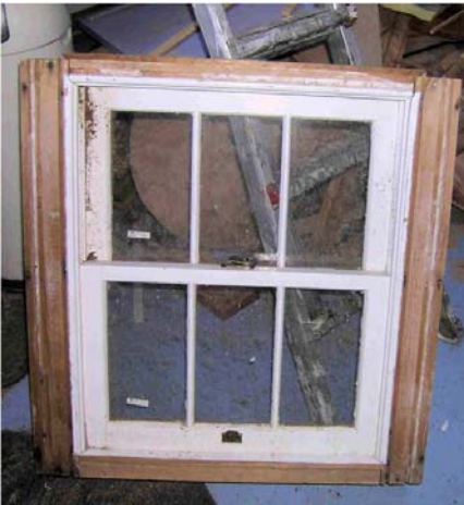
Old window with closed counter weight pockets
