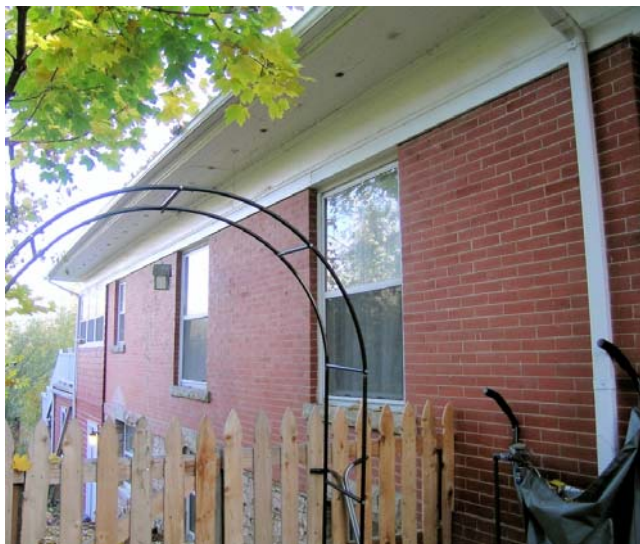
Figure 2-4. Northwest Elevation (The closest 3 windows were chosen for retrofit)
