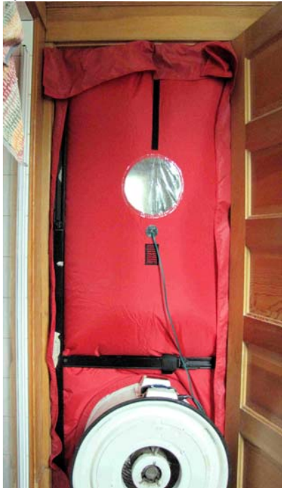
Figure 2-6. Blower Door Installed in Bathroom Doorway
