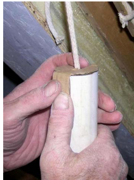
Cardboard in place over PVC tube
