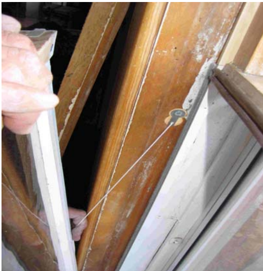
Figure 3-6. Installing spring
