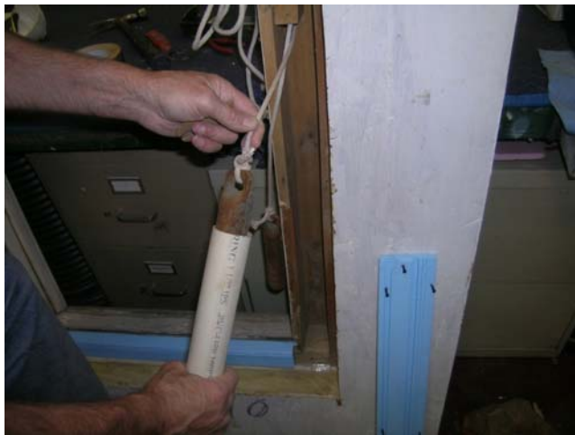
Sliding counter weight into PVC tube
