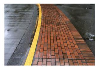
Photo 3.7. (upper left) Example of asphalt paving meeting brick sidewalk.
