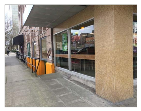
In each of these three examples, the original storefront assembly was replaced with a contemporary version that is not harmonious with the building's historic character. The proportions and materials are out of place. The alterations to the Horseshoe Saloon also resulted in a loss of visual transparency.
