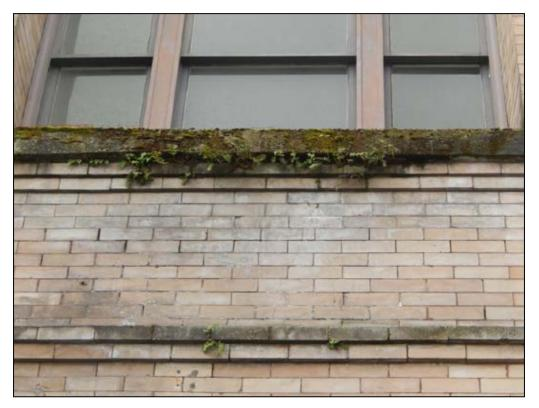
Stone trim and details introduce another color and texture to a building façade. Stone is often used as a window sill or lintel, string course, or cornice. The examples pictured here are showing problems resulting from water damage.
