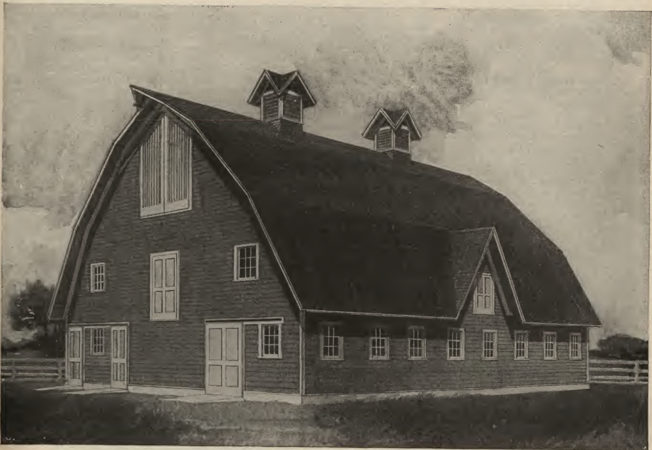
EXTRA WIDE HAY BARN WITH CYCLONE-PROOF DOUBLE-GAMBREL ROOF
