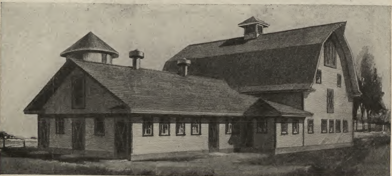
LARGE BARN WITH ONE-STORY COW STABLE ADDITION
