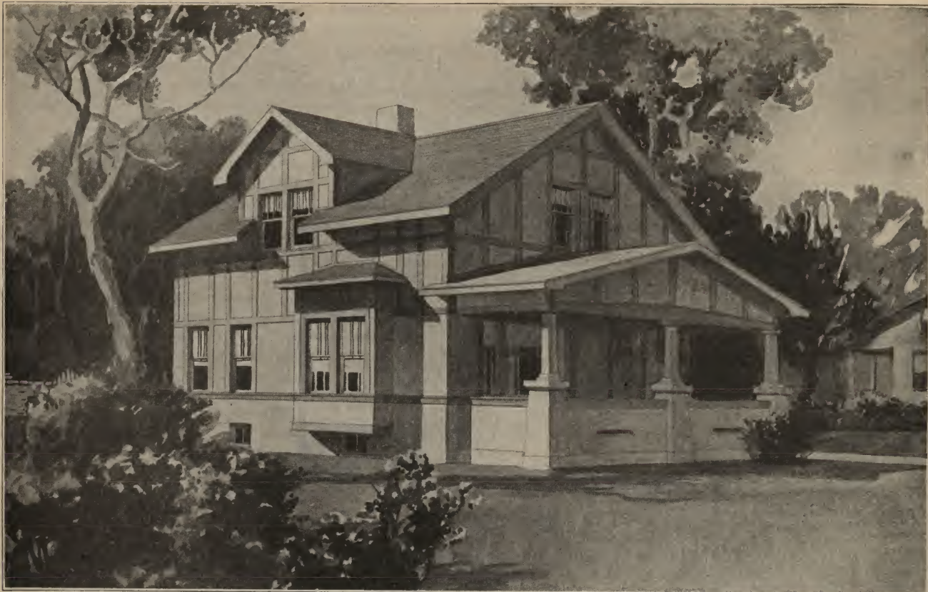
Artistic six-room stucco residence with English half-timber paneling. Size, 28 by 33 feet. We can furnish complete set of blue-printed working plans and typewritten specifications for only $8.00 per set. Blue prints consist of basement plan; roof plan; first and second floor plans; front, rear, two side elevations; wall sections and all necessary interior details. Specifications consist of twenty-two pages of typewritten matter. Ask for Design No. 6544L.
