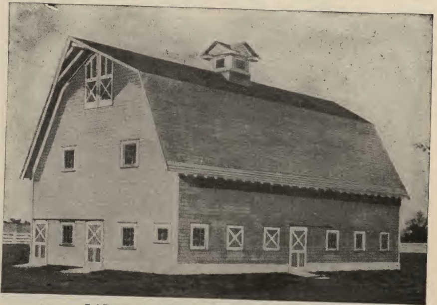
LARGE GAMBREL ROOF HORSE BARN
