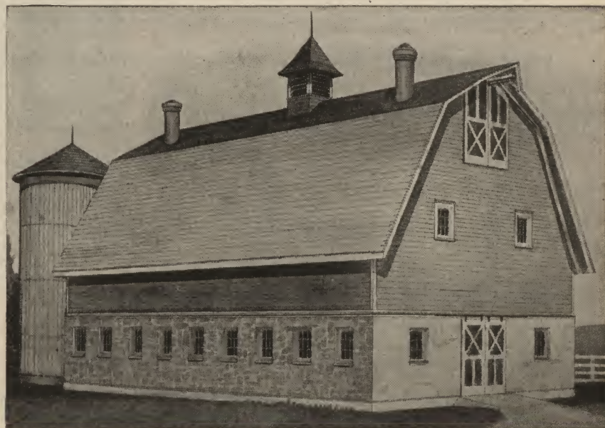
SIXTY BY THIRTY-SIX FOOT BASEMENT BARN
