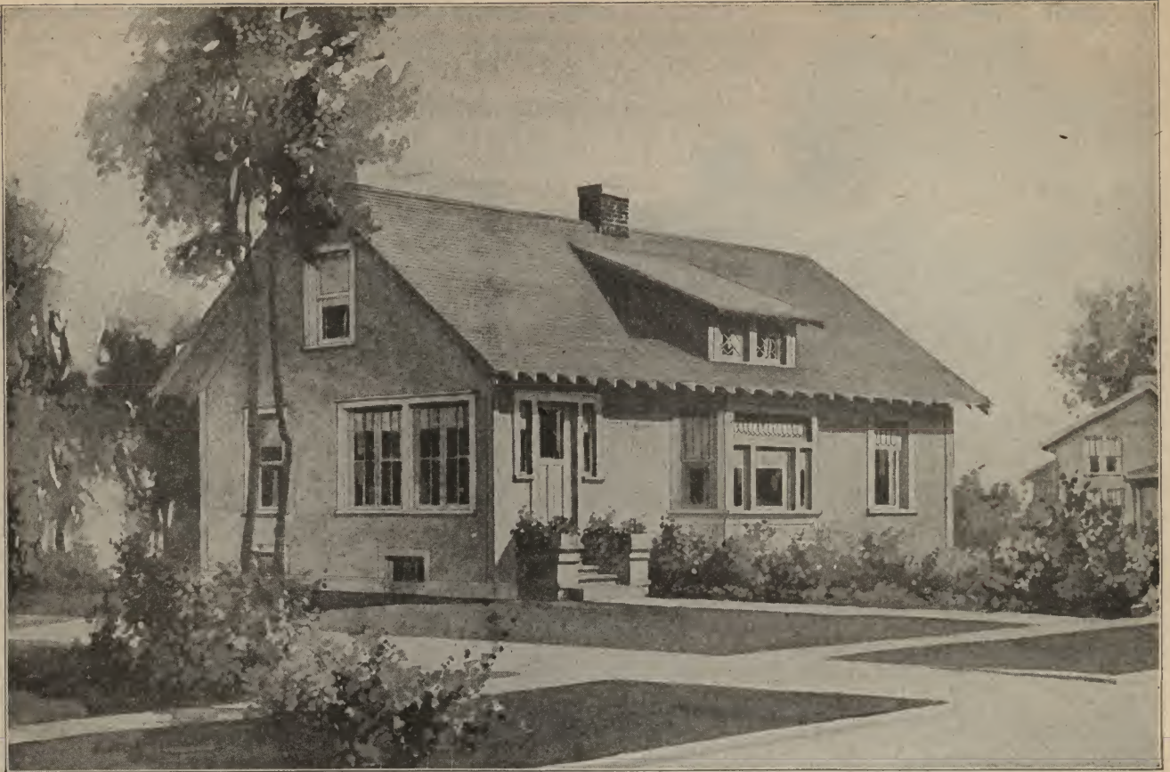
Cozy little cement bungalow containing five rooms. Size, 26 by 44 feet. We can furnish complete set of blue-printed working plans and typewritten specifications for only $6.00 per set. Blue-prints consist of basement plan; roof plan; first and second floor plans; front, rear, two side elevations; wall sections and all necessary interior details. Specifications consist of twenty-two pages of typewritten matter. When ordering, ask for Design No. 6558L.
