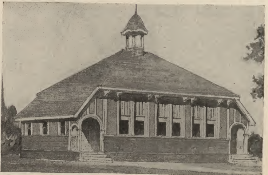
A One-Room Country School of Modern Design and Arrangement.
