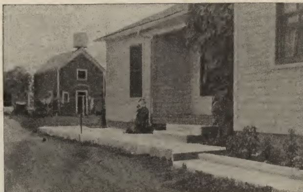
Concrete Put to Effective Use in Several Different Ways on Farm of N. A. Rasmussen, near Oshkosh, Wis.
