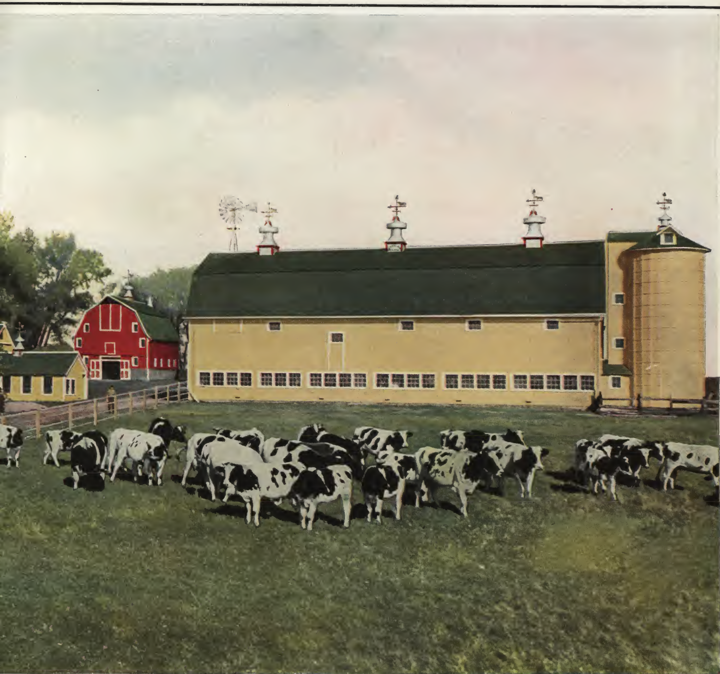
farm buildings equipped with a ventilating system planned for each one individually.
