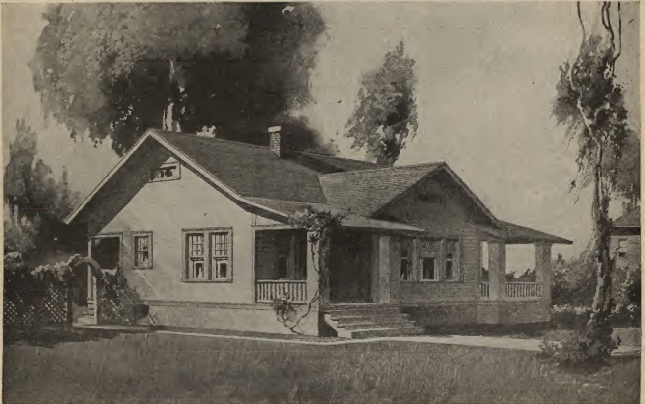
Special six-room bungalow. Size, 46 feet 6 inches by 45 feet 6 inches. We can furnish complete set of blue-printed working plans and typewritten specifications for only $10. Blue-prints consist of basement plan; first and second floor plans; front, rear, two side elevations; wall sections and all necessary interior details. Specifications consist of twenty-two pages of typewritten matter. When ordering, ask for Design No. 6567L.
