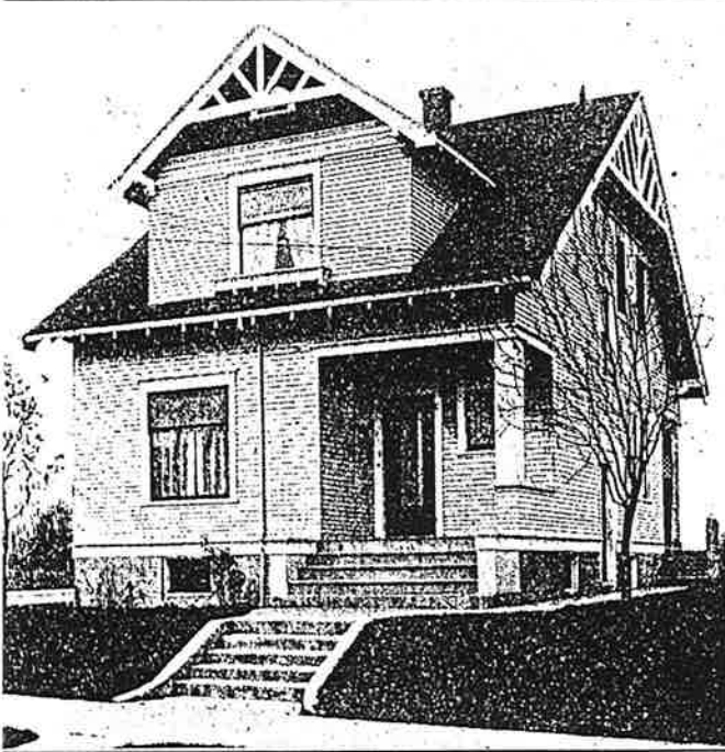
Front view of house No. 601
