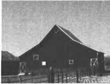
Albert Nelson Farmstead barn (1910), Kittitas County
