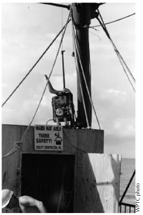
**Figure 35.** This motorized chair was used to hoist workers as they removed paint from the cast-iron columns at the Sand Key Lighthouse. The chair's motor is attached to a hoist, so the chair actually climbs a cable that has been strung alongside the column.
