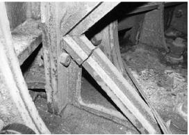
**Figure 18.** The internal structural skeleton of this lighthouse is cracked because of overloading possibly
