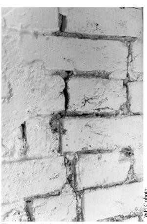
Figure 21. Detail of eroded pointing.
