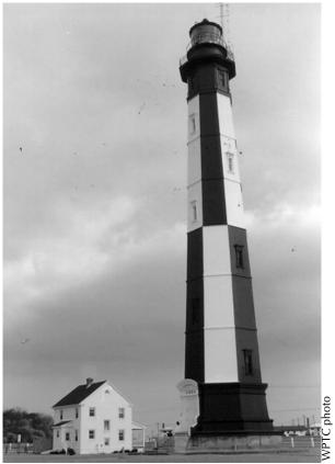
**Figure 4.** Double-wall, cast-iron, first-order 163-foot-tall coastal tower at Cape Henry, Virginia.
