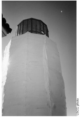
**Figure 22.** View of the lighthouse scaffolding covered with shrink wrap to contain all hazardous materials and protect workers from severe weather.
