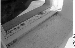
**Figure 26.** This steel casement window frame was not sealed properly and as a result has begun rusting from the inside out.
