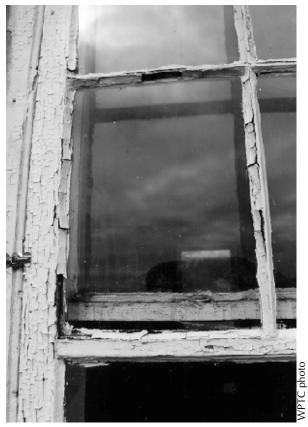
**Figure 7.** Deteriorated glazing putty and peeling paint on a multilite wood sash.
