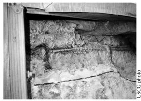
**Figure 28.** Close-up of the damaged concrete gallery deck after the loose concrete has been removed and before the damaged concrete was repaired using pressure-injected epoxy grout.
