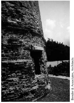
**Figure 26.** View of the lower tower window; note the depth of the brick deterioration at the window openings. The face of the protruding granite lintel above the window opening represents the face of the original wall.
