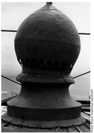
**Figure 8.** Despite the fact that this first-order lantern ventilation ball has been repaired several times, it still provides adequate lantern ventilation.
