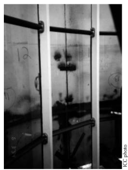
Figure 7. Inside the lantern room, the mullions have been reworked and reattached to the stiles. New stainless steel bolts have been used to prevent corrosion and teflon tape has the used as a gasket between the bronze and the cast iron. Teflon washers also separate the bronze from the stainless steel bolt.
