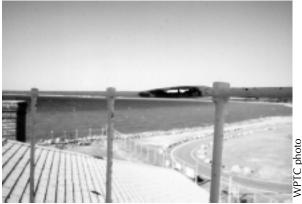
**Figure 26.** Detail of handrail that is being deformed by rust-jacking.
