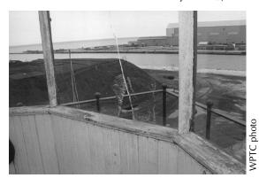
**Figure 7.** Lantern glass with holes and/or cracks should be replaced as soon as possible to minimize water infiltration. If immediate replacement is not feasible, the glass can be temporarily patched.
