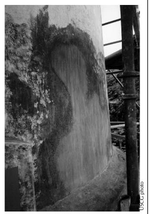
**Figure 27.** The areas where the loose mortar finish coat was removed were repaired with a two-part mortar patch. The final texture on the patch was tooled to match the historic wall surface. The patch was completely invisible after the tower was painted.
