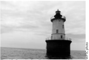
**Figure 3.** Example of an all-cast-iron construction "sparkplug" caisson-style lighthouse.
