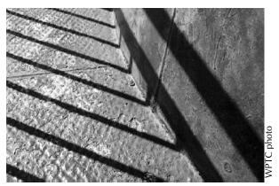
**Figure 25.** The seams between the deck and wall plates of this lighthouse were not properly sealed; as a result the areas collected water and began to rust.
