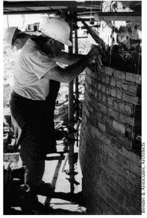
**Figure 28.** Here a mason is implementing repairs to the exterior wall. The missing bricks were replaced with inkind materials: the bricks match the historic bricks in size shape and strength. The mortar joint sizes are also being made to match the historic in size, color, and texture, as demonstrated in this photo. The vertical strings over the brickwork define the wall plane, so when the mason places the bricks, they maintain the taper of the conical tower.
