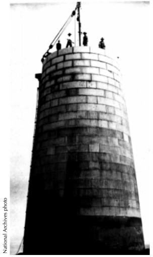
**Figure 31.** Work on Minots Ledge Lighthouse as it progressed just above the entrance level which is visible on the left. The tower below this level was essentially solid.
