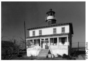
**Figure 2.** Example of a keeper's quarters fitted with a prefabricated cast-iron-and-steel lantern.
