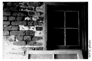
Figure 11. Detail of severely eroded brick and painting.
