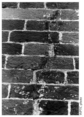
**Figure 15.** Cracks such these in a sandstone lighthouse should be monitored for movement prior to treatment.
