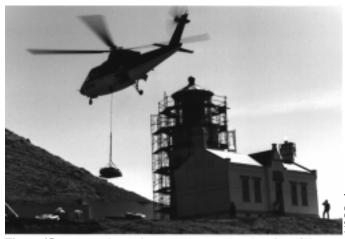
**Figure 45.** *Staging the work.* Note the temporary location of the auxiliary light on the fog signal building chimney.
