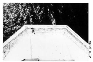
**Figure 8.** View of a wood-framed lighthouse roof; the arrow indicates where a large hole (approximately 2 by 4 inches) is present in the built-in gutter system. Water entering this hole has caused extensive damage to the interior wood framing members and wood interior wall paneling.
