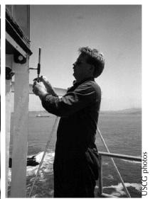
**Figure 37.** After drilling, threads were cut into each hole using a hand-operated tap.
