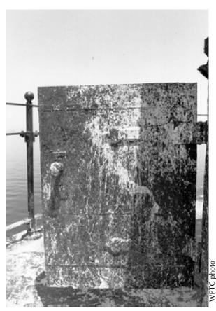
**Figure 28.** Surfaces such as this sheet-steel-covered parapet door that are covered with seagull guano should be thoroughly cleaned before mothballing and should be checked and cleaned once a year during the mothballing period.
