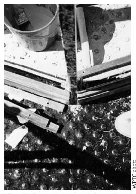
**Figure 12.** Detail of the bronze sill when the lower mullion is removed; the fastener is re-tapped and the cast-iron column is treated with a rust converter. Note that the bronze astragals have been cleaned and are ready to accept the glazing system.
