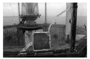
**Figure 6.** An acceptable temporary lantern glass repair made using a small piece of sheet metal and caulking.
