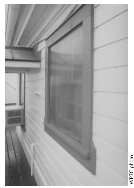
**Figure 13.** This image shows a Class I paint condition: virtually no deterioration, only some soiling and possible salt buildup resulting from the open-water location of the lighthouse.
