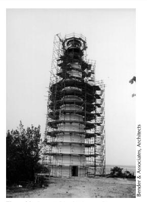
Figure 24. Cape Florida Lighthouse with scaffolding used during the 1996 restoration. The white coating on the tower is the lime mortar wash applied to help protect the damaged brick and to restore the tower to its 1846 appearance.
