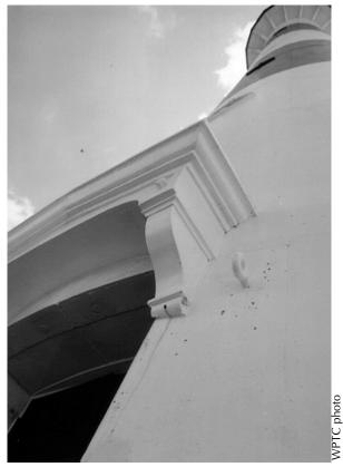
**Figure 45.** Within three months after painting, the rust began to bleed through this weep hole on the bottom of this pediment bracket. Two lessons are to be learned from this condition: 1) keep weep holes open to allow any water that may have entered the casting to escape, and 2) keep joints around applied castings sealed; apparently this was not done and water has entered the hollow cavity of the pediment, causing rust to form inside.
