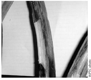
**Figure 13.** Close-up of a dutchman repair (light-colored wood used to mend a window muntin).
