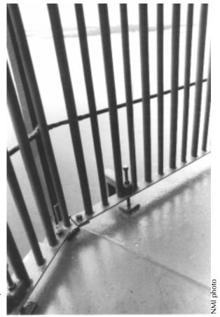
**Figure 26.** Note how the cage is clamped to the gallery deck, minimizing any impact on the structure's original fabric.
