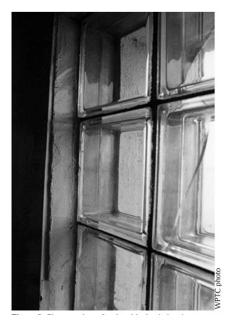
**Figure 8.** Close-up view of a glass-block window in a concrete lighthouse. The joint where the glass block meets the concrete wall should be caulked to prevent moisture infiltration.
