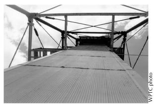
**Figure 9.** If the exterior of the wooden tower has been covered with another sheathing material like this corrugated metal, all joints in the exterior sheathing should be made completely weathertight; at this particular lighthouse, deterioration of interior wood framing members was caused by moisture infiltration.
