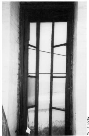
**Figure 11**. Example of a metal casement window in a lighthouse dating from the 1870s
