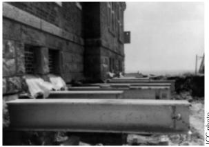
**Figure 18.** Large cross steel beams are inserted into the cut opening to form part of the grid that will carry the building.
