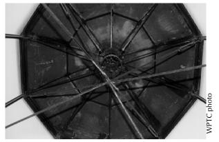
**Figure 21.** The diagonal tension rods in this empty lantern were installed to brace the lantern against lateral loading caused by high winds.
