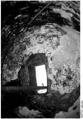
**Figure 4 (left).** Extensive interior finish deterioration in a lighthouse that had holes in the roof which were not repaired.
