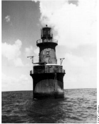
**Figure 7.** Sabine Bank Lighthouse with caisson foundation in Texas.
