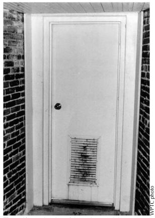
**Figure 10.** Interior view of the modern metal door at the Ocracoke Lighthouse before its replacement; corrosion like this should be removed and the affected areas treated with a rust-inhibiting coating system.
