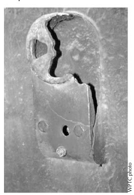
**Figure 14.** Nearly 30% of this ventilation shroud has been lost to two forms of abrasion: first, sand or grit blasting abraded away a majority of the material; second, human touch has smoothed the once rough surface.
