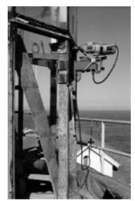
**Figure 35.** Jig used to bore holes in the gallery bracket tenons.
