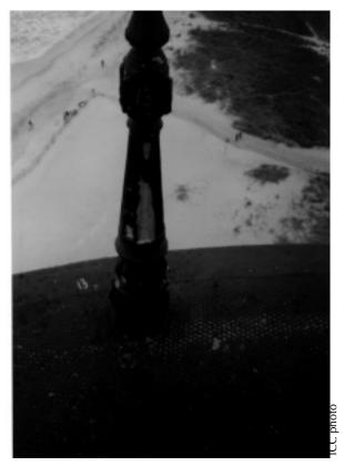
**Figure 14.** The handrail assembly has been removed and the ornate cast-iron post is ready for removal.
