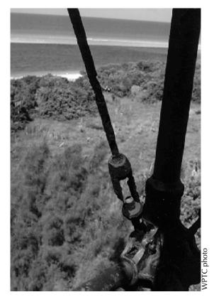
**Figure 16.** As corrosion attacked this steel turnbuckle, wind and airborne sand eroded away the flaking rust.
