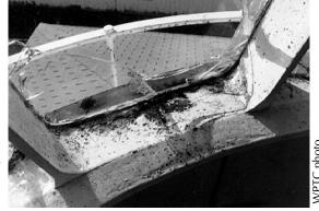
**Figure 12.** The glass in this lantern has been cracked by the rust-jacking that is occurring along the iron frame.
