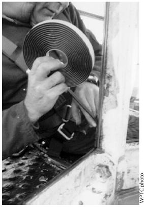
**Figure 15.** The polybutyl sealant tape was placed on all receiving surfaces on the plane of the interior face of the glass and on the inside faces of the exterior astragals.
