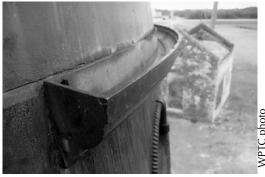
**Figures 23 and 24.** Two types of gutters found on iron lighthouses; the gutters must be in proper working order and checked regularly during the mothballing period.
