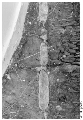
**Figure 32.** This sheet-copper-covered lantern gallery deck has been repaired several times by soldering sheet copper patches over the holes. This method of repair, if performed properly, greatly increases the life span of the roof covering.
