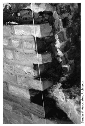
**Figure 27.** View of repairs being made to the exterior wall. A new brick wythe is being installed where bricks were missing, using mortar that matches the strength of the new and historic bricks. Masonry anchors are used to attach the new wythe to existing wall. The deteriorated mortar joints in the extant wall were repointed with a matching mortar mix.
