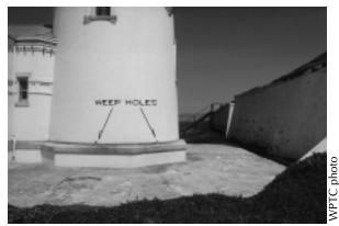
**Figure 12.** Typical masonry lighthouse weep hole locations. Each weep hole provides drainage for each individual cavity within the masonry wall.
