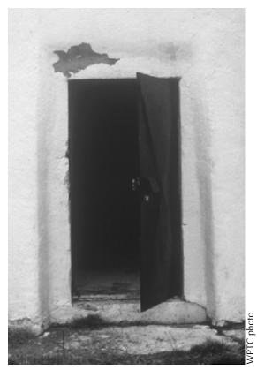
**Figure 13.** Site-built steel door at the Turkey Point Lighthouse; this solution was chosen because of the remote location and repeated break-ins. Note exterior stiffeners and shroud over the hasp and lock.
