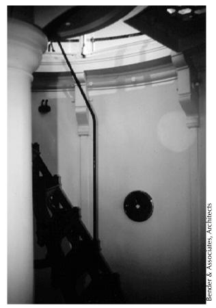
Figure 38. Service room bracket after chemical cleaning.
