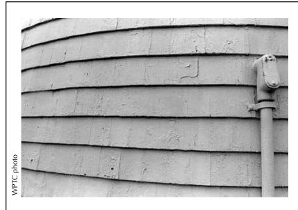
Figure 15. View of Class III paint condition: in this case the cracking, peeling, and alligorating have been caused by excessive paint layer build up.
