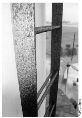
**Figure 11.** Detail view of a steel ladder that has been uniformly attacked by corrosion.
