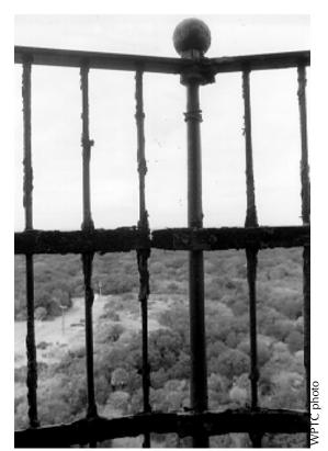
**Figure 13.** View of a steel railing where corrosion has occurred in distinct locations either because of variations in composition or localized failure of the coating system.
