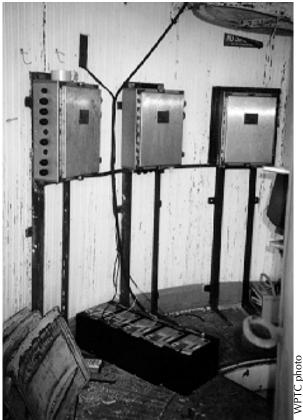
**Figure 33.** To minimize damage to historic wood beadboard panelling, these new panels should have been installed on a sheet of plywood attached to the historic wood beadboard panelling in four locations. These batteries stored on the floor should be in containment boxes in case the batteries leak.
