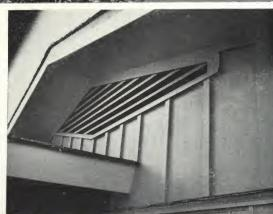
Bedrooms are cooled in summer by big attic fan circulating air through ceiling louvers (right). In winter, Exterior plywood sheets (right, below) close louvers as ventilation for coolness is not required, although some circulation of air in attic is prerequisite to good construction. Note interesting texture contrast between smooth plywood soffits and plywood and batten siding.
