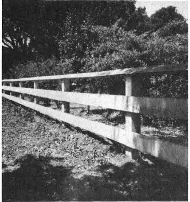
Setting the top guard rail at an angle keeps children from walking fence, makes it stronger, and protects ends of posts
