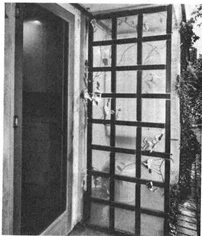
Harold Bradley, Design; Jerry Anson, Photo Strips of one-by-two-inch redwood arranged in an interlocking pattern of 10-inch squares over plastic-covered wire screen
