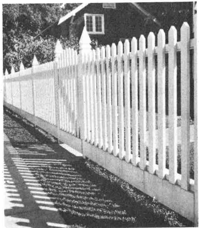
White picket fence is trim and friendly. Here the design of post heads illustrates one of many possible variations
