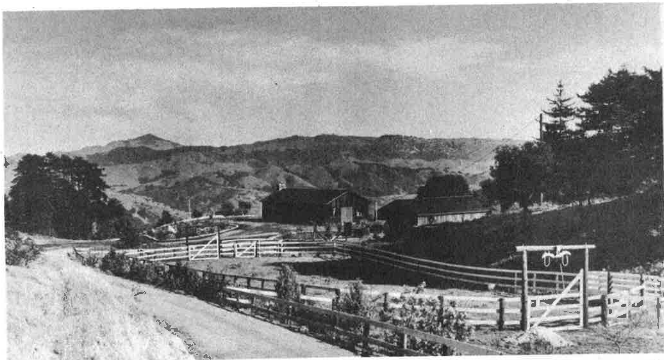
Above: Rail fencing gracefully follows the contours of the countryside. Whitewashed boards nailed to round, peeled posts
