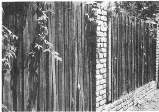
Handsome variation of rustic picket fence makes use of rosy bricks in low wall and posts spaced about 6 or 7 feet apart
