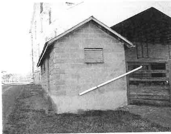
Figure 13. Milk house, Franklin County, Pennsylvania, c. 1935. This milk house has decorative rock-face concrete block on the side facing the road, while the remainder not visible to the public is made of simple concrete block. Photograph by the author, 2009.
