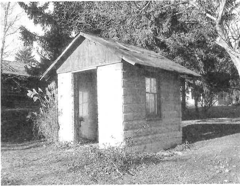
Figure 21. Milk house, Upper Brush Valley Road, Centre County, Pennsylvania, c. 1925, west and south elevations. This diminutive milk house was carefully built of rock-face concrete block with corner quoins. Photograph by the author, 2011.
