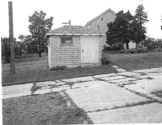
Figure 14. Milk house, Lebanon County, Pennsylvania, c. 1920. This milk house is constructed of yellow hollow-tile block, and its hipped roof has decorative wood trim. Photograph by the author, 2009.
