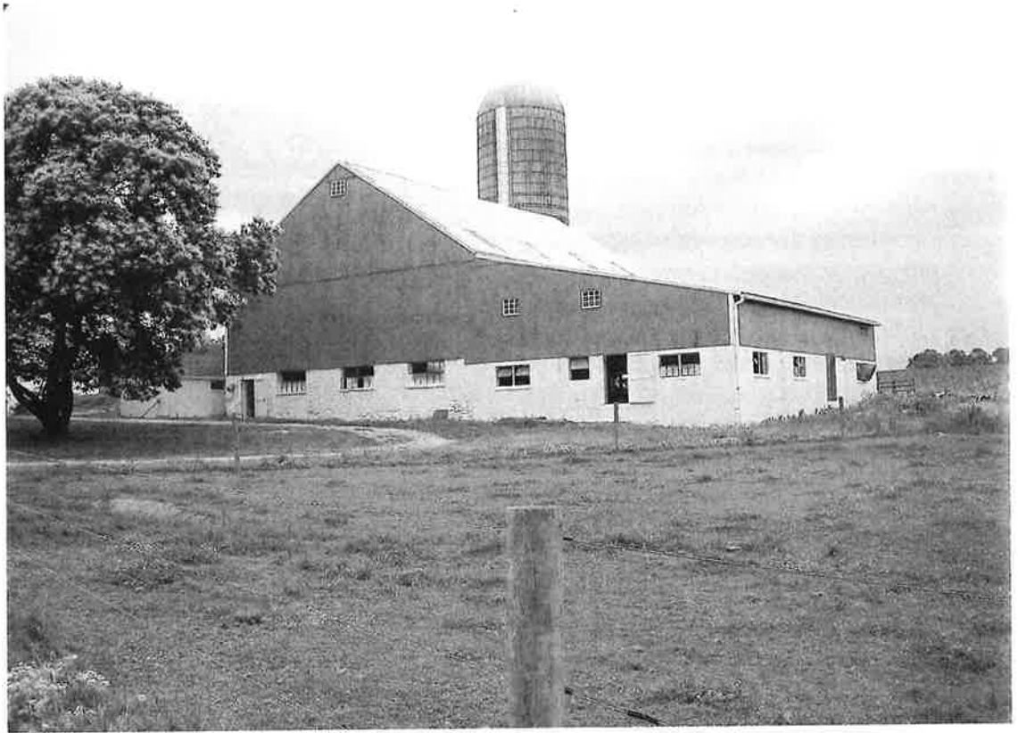
Figure 9. Renovated barn, Chester County, Pennsylvania. Originally, this nineteenth-century barn probably had the extended posted forebay characteristic of southeastern Pennsylvania. In the mid-twentieth century it was renovated for dairying. The forebay was enclosed with a concrete-block wall with windows inserted; stables were concreted; and tilting metal windows were inserted into the original stone foundation wall. Photograph by the author, 2010.
