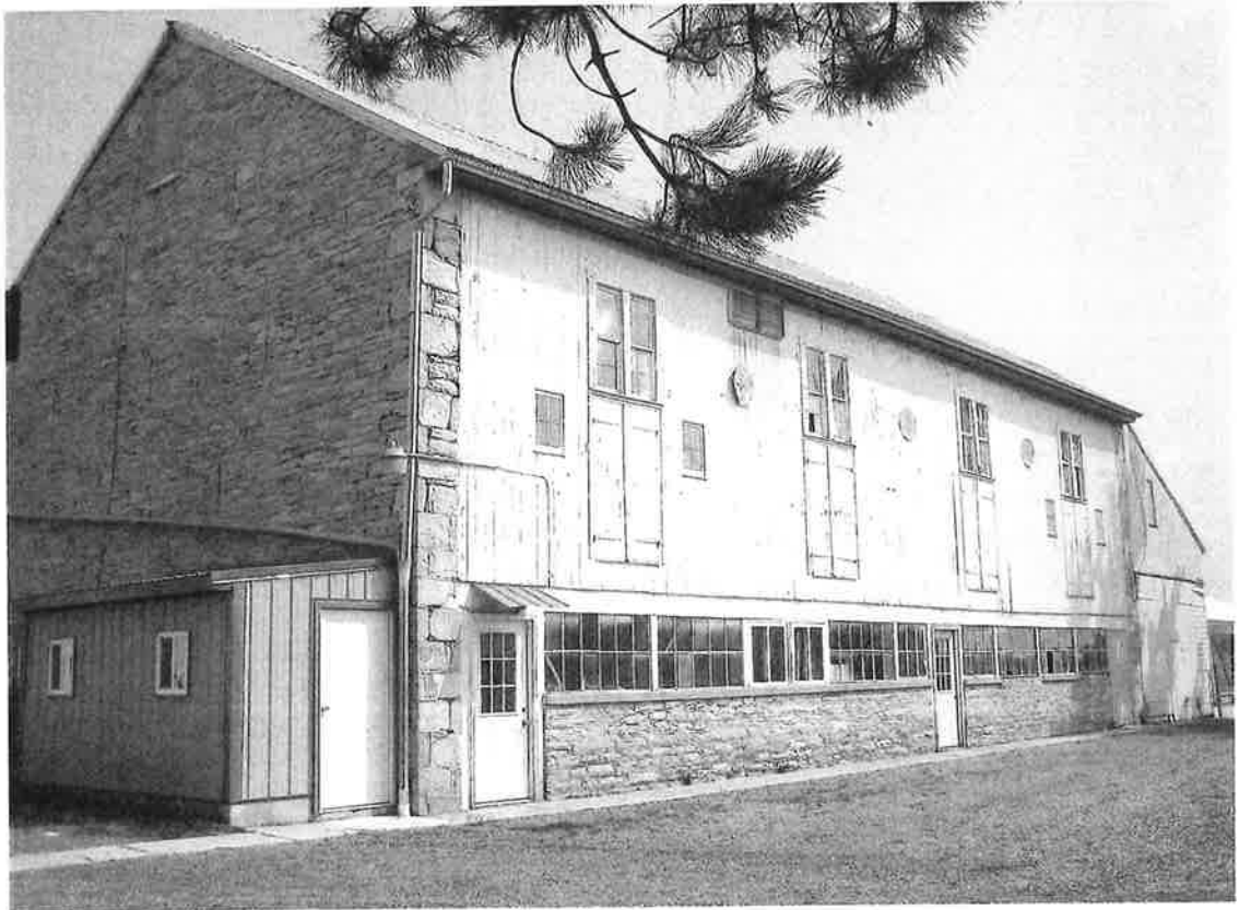
Figure 10. Renovated barn, Lebanon County, Pennsylvania. The original portion was built around 1850. About 1925 the forebay was enclosed with a stone wall with long strips of windows. Photograph by the author, 2009.
