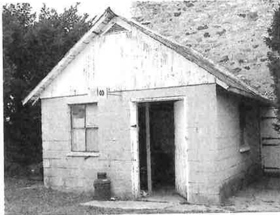
Figure 12. Milk house, Chester County, Pennsylvania, c. 1940. This concrete-block milk house has projecting window sills, mullioned windows, and a triangular vent in the gable peak. It abuts a much earlier barn. Photograph by the author, 2010.
