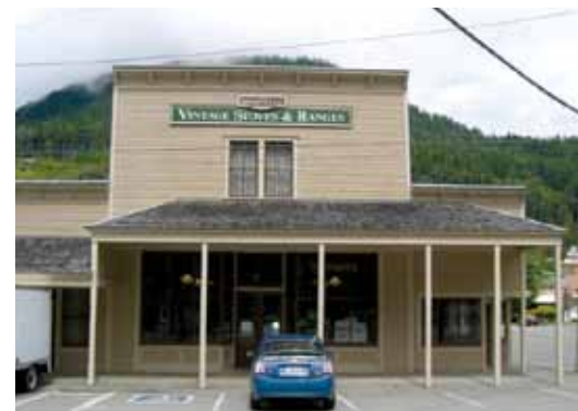
Maloney's Store (1893), Skykomish Top: Historic View c. 1905 Middle: Store c. 1993 Bottom: After rehabilitation, 1996
