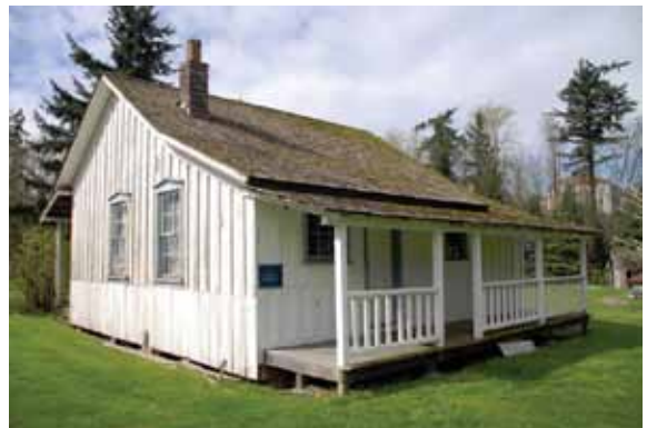
Pacific Coast Coal Company House (c. 1880), Newcastle
