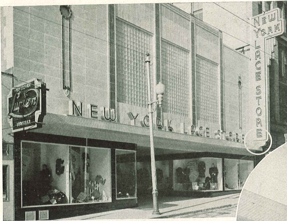
Above: Cornice as illustrated shows a combination of no. 8 and no. 9 sections. No visible fastening necessary.
