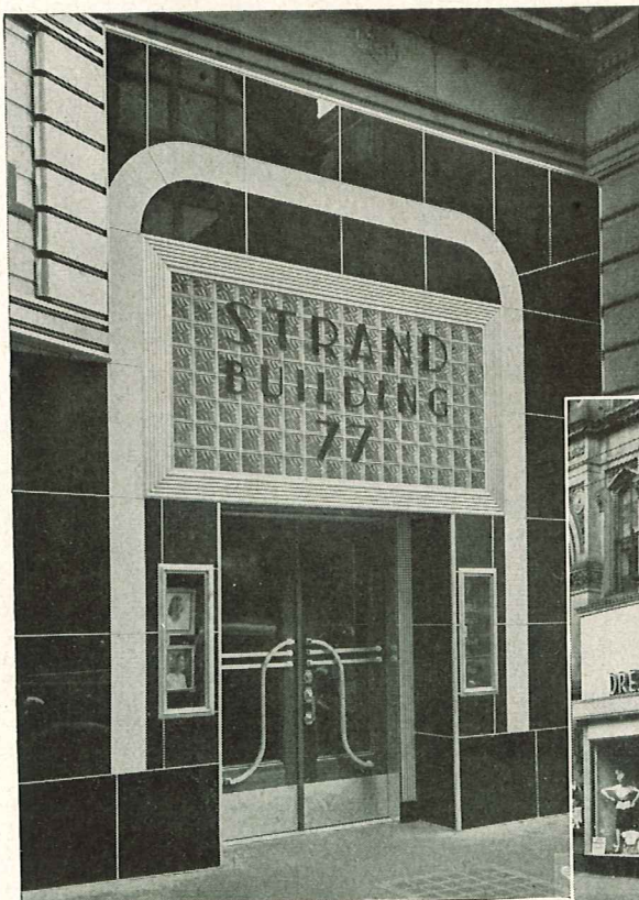
Above: Glass block panel framed with a combination of no. 22, no. 23 and no. 24. Display cases fabricated from a combination of no. 1 and no. 12.
