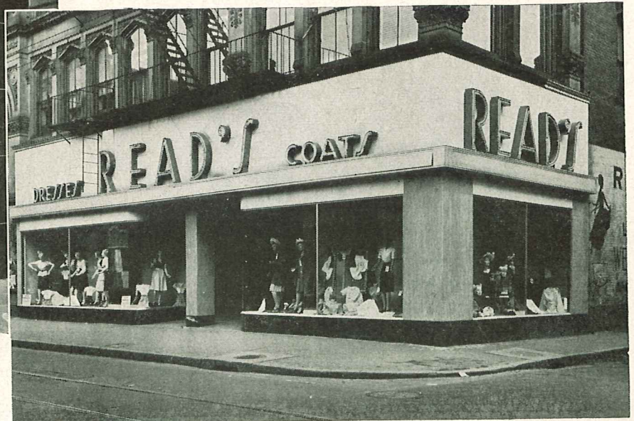
Below: No. 189 concealed awning hood cover, shown partly open, made from a combination of no. 3, no. 8 and no. 12.
