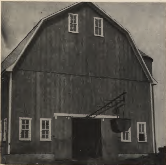
Swinging Crane or Boom Attached Directly to the Barn
