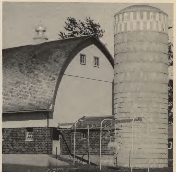
Installation Using Steel Arch Track Support
