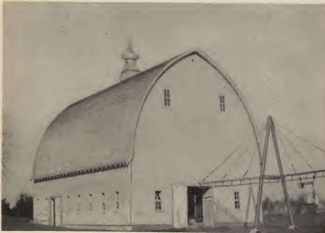
Bridge and Crane Installation Using a Steel "A"
