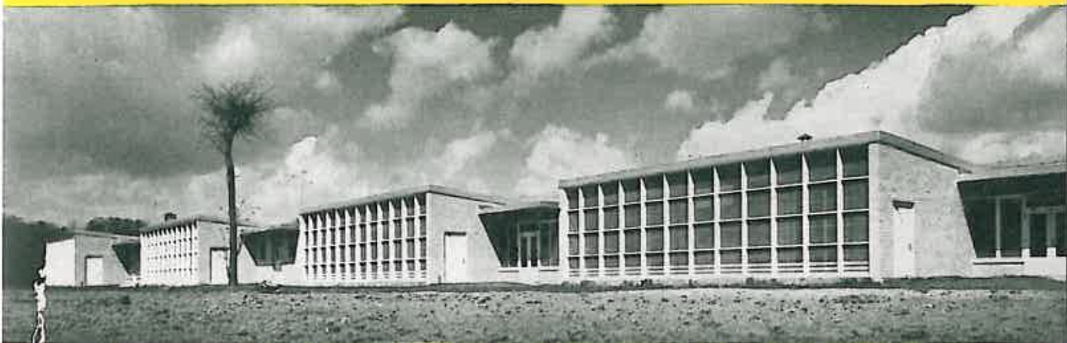
South elevation features hospital's "cottage" units. Sliding glass doors behind screened porches can be opened for fresh air.
