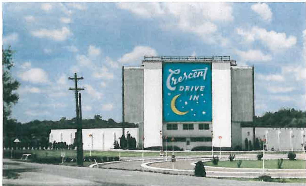
PPG Cementhide Rubberized paints (now available in over 100 colors) were used to decorate Crescent Drive-In, Nashville, Tenn.
