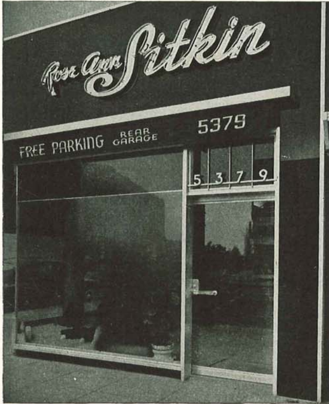
Products used: Carrara; Polished Plate Glass; Pittco Metal. Architect: Stiles O. Clement.
