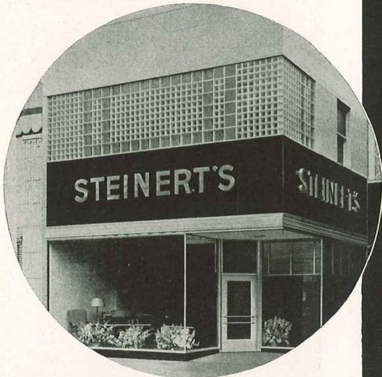
Products used: Carrara; Polished Plate Glass; 6" and 12" Argus PC Glass Blocks; Pittco Metal. Architects: McClintock & Craig.
