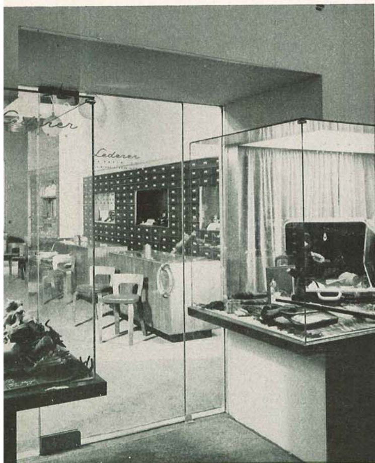
A free-standing Herculite Door without separation between the door and the adjacent Herculite Panels. The clarity of vision afforded by this treatment is well illustrated by the view obtained through the display windows, the door, and the side panels. Victor Gruenbaum, associate designer, Morris Ketchum, Jr., architect.
