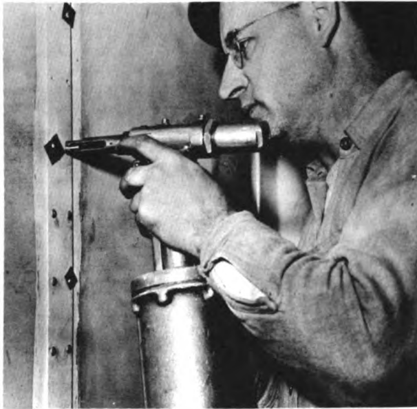
Fig. 3.21—Riveting porcelain enamel coated sheet.
