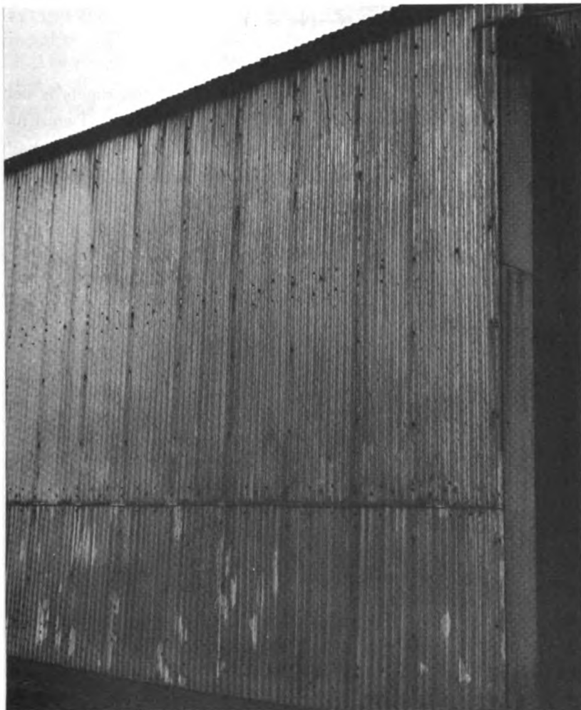
Fig. 4.13—Both the interior and the exterior of the ore-thawing building receive as severe abuse as any building, being continually wet and exposed to considerable dirt. No visitor to the building can resist rubbing a small area of the porcelain enamel siding—witness the several rubbed areas on the bottom panels, exposing bright, clean, unaffected enamel.
