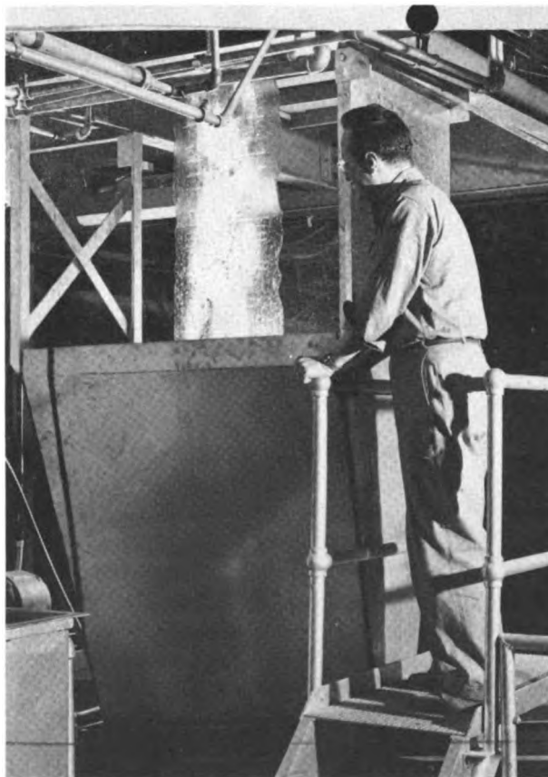
Fig. 1.34—From the rolls above, the molten glass drops onto a vibrating conveyor at a lower level.
