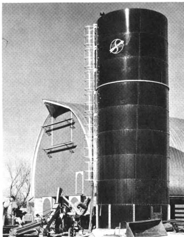
Fig. 1.14—Typical porcelain-enameled silo installation. The structure is porcelain enameled inside and out, thereby providing an acid-resistant, abrasion-resistant structure which will require a minimum of maintenance.
