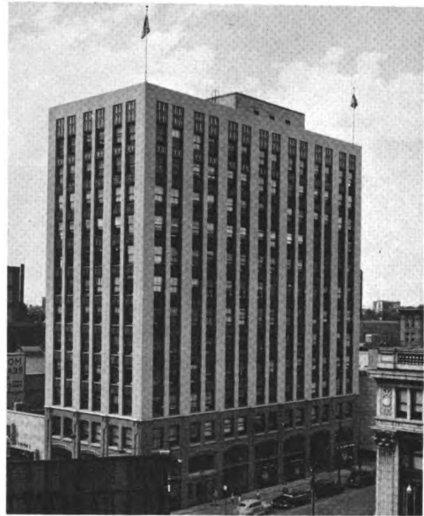
Fig. 1.4—Built in 1926, the Security Building in Denver, Colorado was completely modernized 25 years later. Roland L. Linder and Associates, the architects, selected acid-resistant architectural porcelain for the exterior "face lifting." The project required the stripping back to the structural members of the 12-story building and the removal of approximately 900 tons of brick and terra cotta. The total weight of the "face lifting" architectural porcelain was only 30 tons. The pastel green, stipple finish was pleasantly contrasted by aluminum-colored caulking compound.
