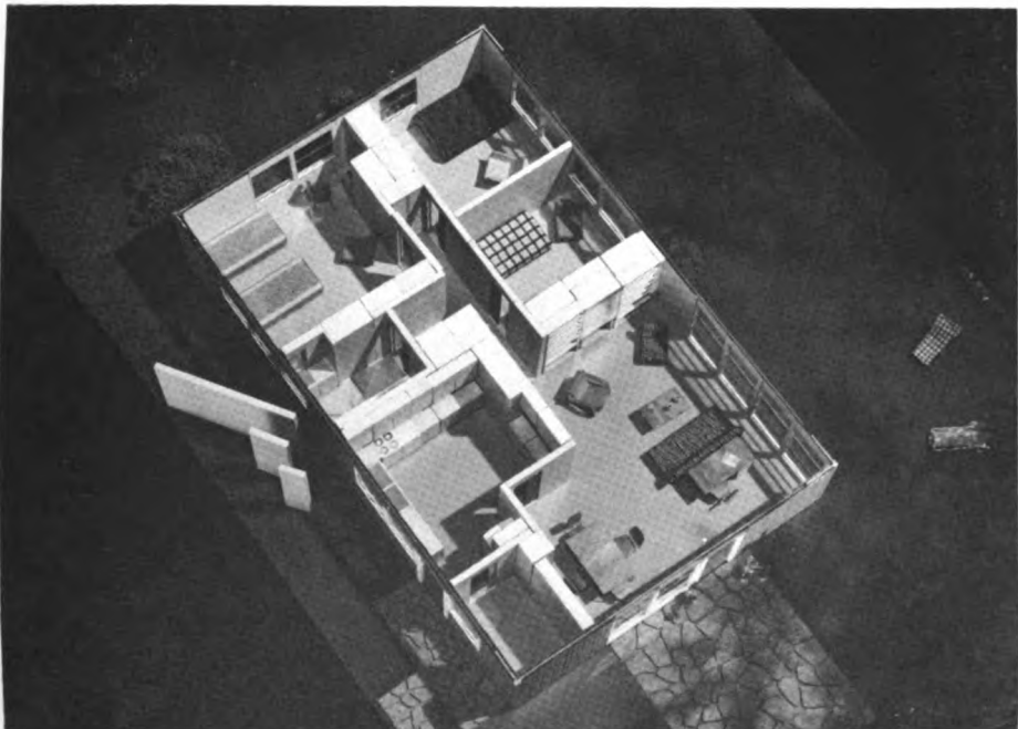
Fig. 2.14—Model of proposed 1950 three-bedroom Lustron House. Plan view showing use of various interior and exterior components.
