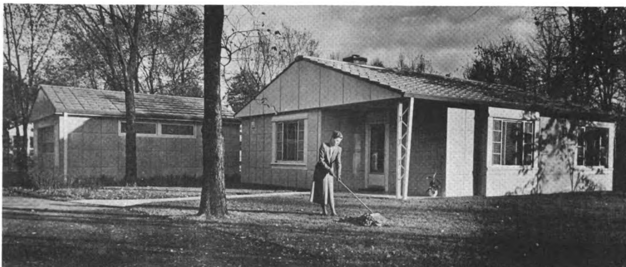
Fig. 2.10—Lustron House, 1949. Porcelain enameled panels used for roof, gable ends, and walls. Wall panels measure two feet square, roof "shingles," one by eight feet. Interior surfaces are also porcelain enameled steel. Purchasers were offered a wide range of integral pastel colors, inside and out.
