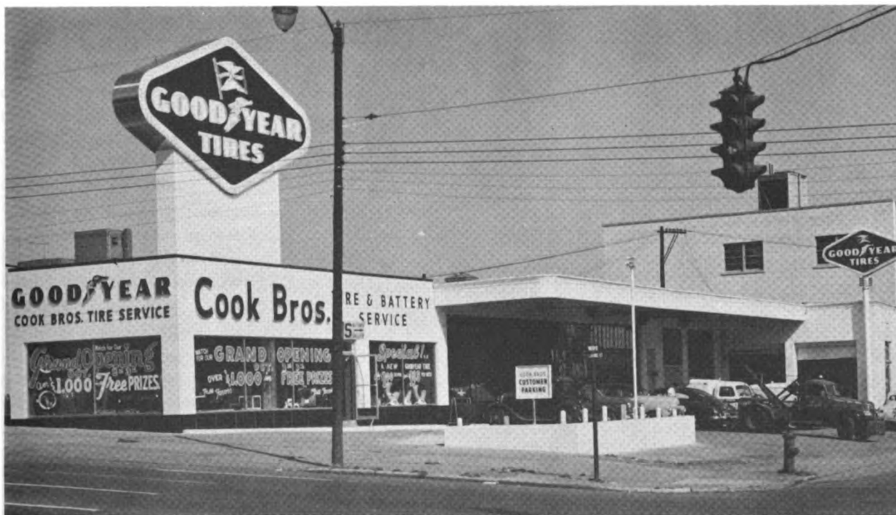
Fig. 4.8—The completed Cook Bros. structure.
