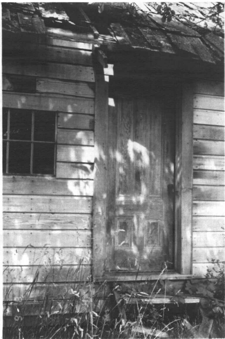
SALVAGED DOOR & WINDOW - STRAWBERRY HILL
