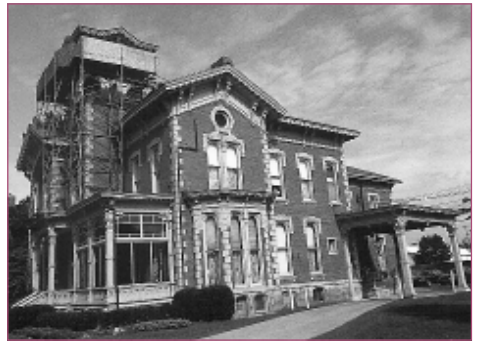
Kalamazoo, Michigan American Red Cross Restoration Project
