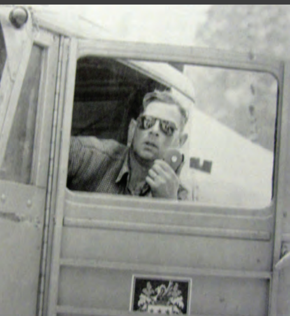
Late 1940s DOT road worker.
