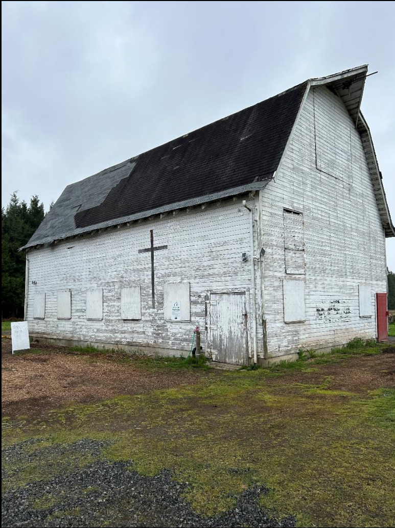
Stevenson - Wilcox Barn, Marysville – 1928
