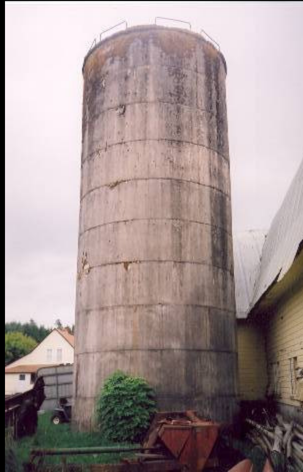
Poured Concrete Silo Cloverdale Farm – c.1935
