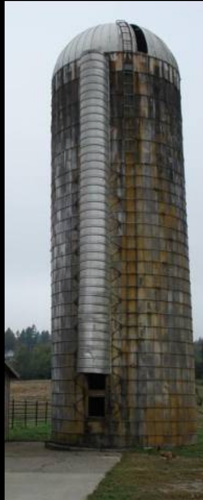
Concrete Stave Silo Zarcrossed Farm – c.1920
