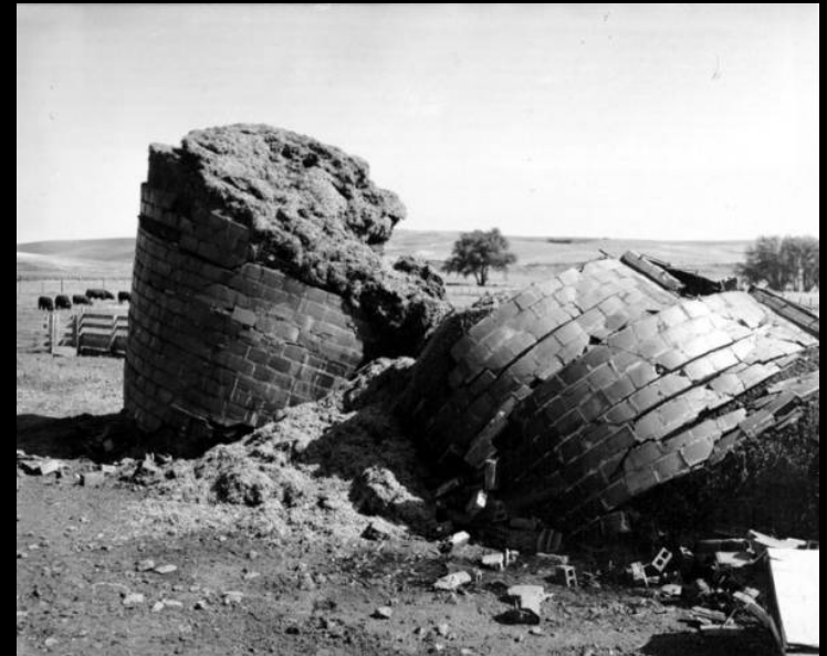
Glazed Tile Silo Whitman Co. - 1920
