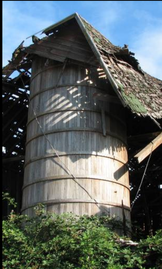
Vertical Wood Stave Silo Clark Co. – c.1900
