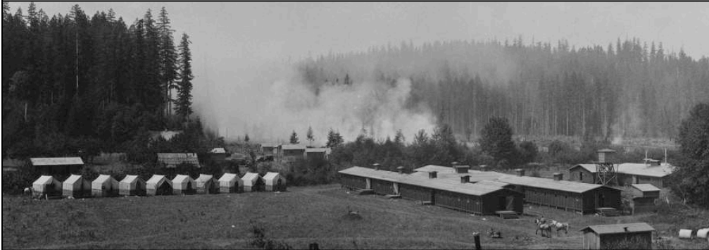
8/8/1923 – Clearing land to build a town.
