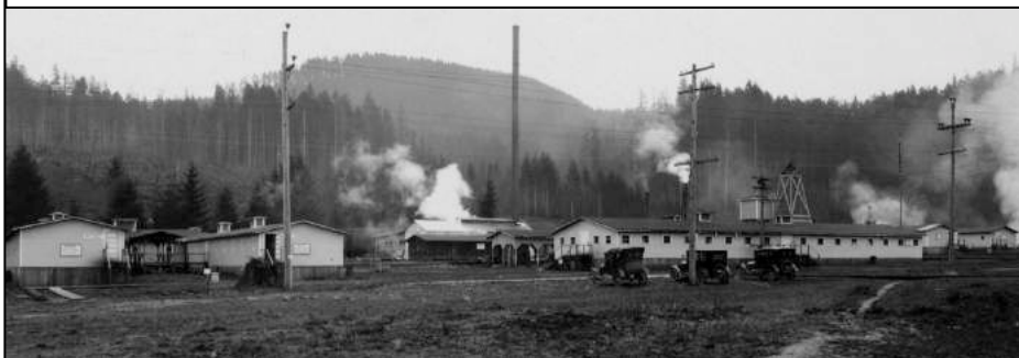
2/2/1926 – Modern steam-heated dormitories for single men employed at Ryderwood. LPL date.
