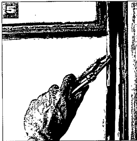
To remove the parting bead, grasp it with locking pliers (5), then work the strip out from the notch in the upper sash meeting rail. Note that the bead may already be weak or worn at this point. Angled ends and a single wood screw secure the weight pocket door (6) and access to the weights.
