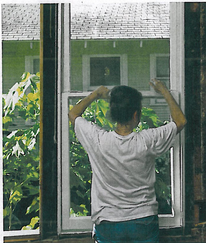
After replacing the top sash and tying on and adjusting the weights, Pam fits the bottom sash into the window.
