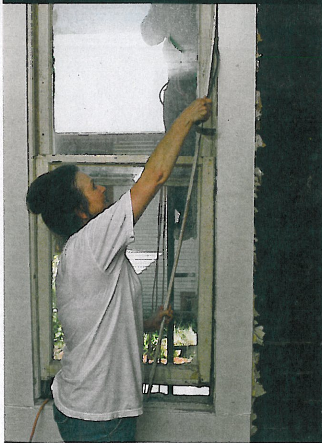
Pam begins the window restoration by removing nails and screws and carefully prying off trim and interior stops.
