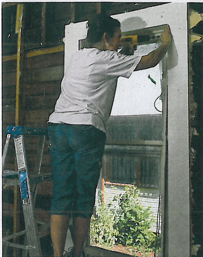
Pam begins the window restoration by removing nails and screws and carefully prying off trim and interior stops.
