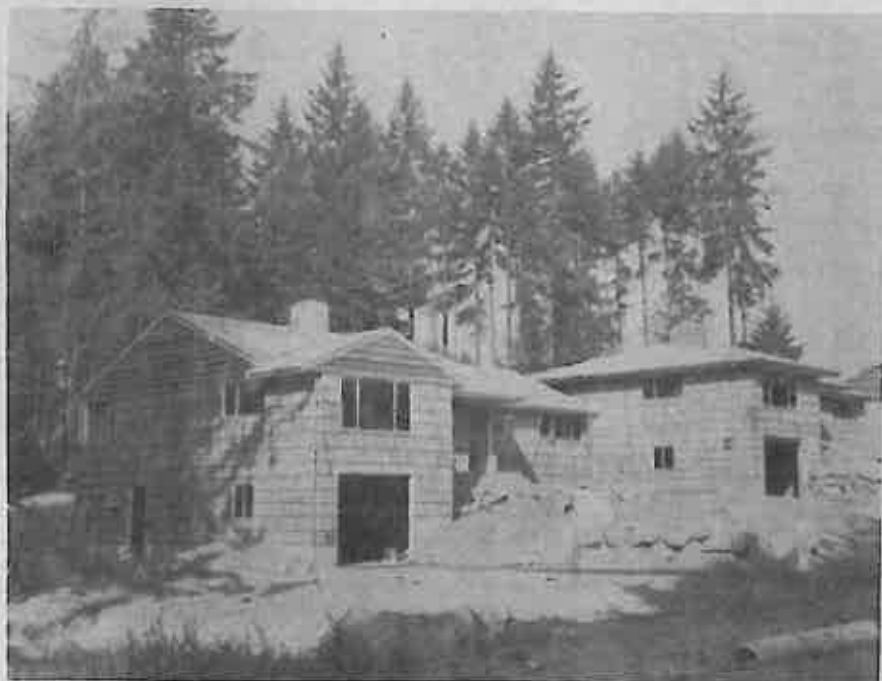
NEW BASEMENT MODEL under construction
