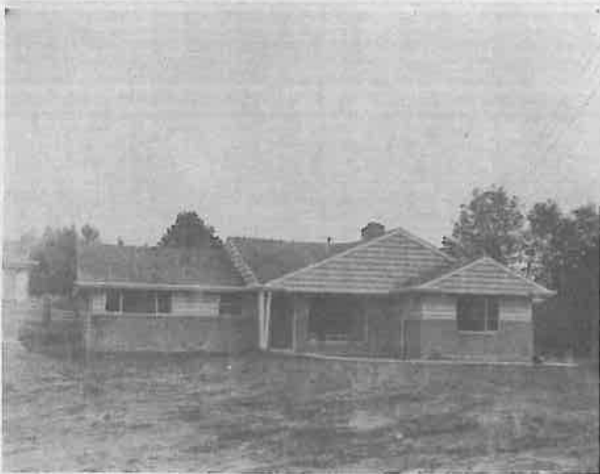
JUST COMPLETED, READY FOR LANDSCAPING
