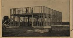
74 Hours' carpenter labor shows the framing of barn apidly nearing completion.
