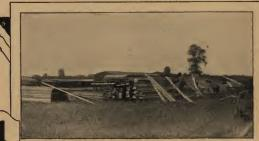
Lumber delivered in random lengths. Time is lost in measuring, cutting and getting material.
