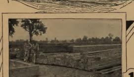
All framing lumber cut to exact length and shape, ready to be nailed in place. No time lost in measuring, cutting and fitting.
