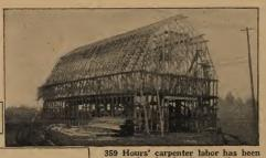
359 Hours' carpenter labor has been spent and only the framing is completed.
