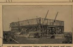
172 Hours' carpenter labor needed to erect and complete the frame to the plate line.
