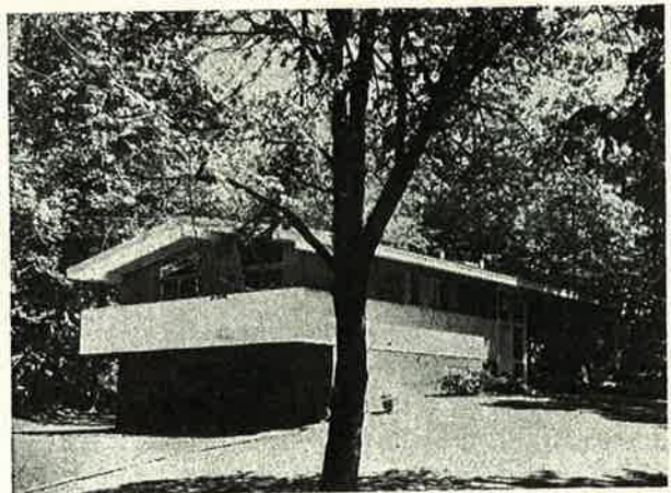
BALCONY and low-pitched roof give a fine contemporary feeling to this Shroder Co.-built house which goes for $33,250 without land; plan is national favorite.
