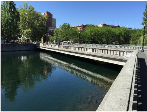
17. South Channel Bridge
