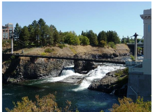
14. South Suspension Bridge
