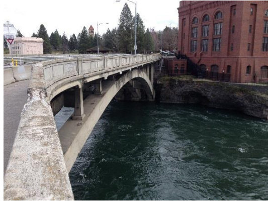
37. Post Street Bridge (Not Eligible)
