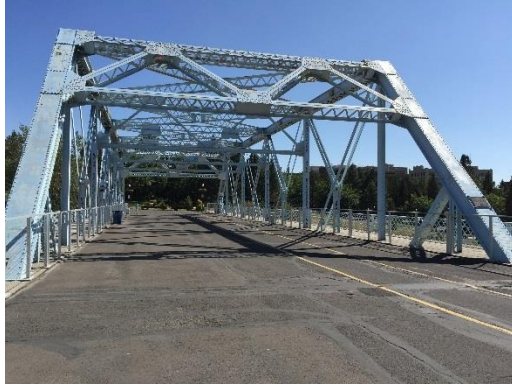
16. Mid Channel Bridge (NRHP-Eligible)
