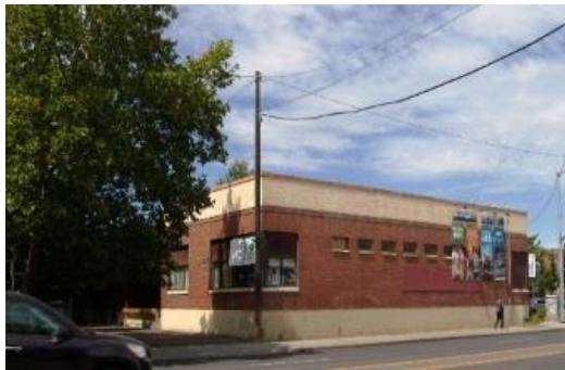
23. Expo '74 Services Building (Not Eligible)
