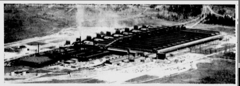
ALUMINUM PLANT More than 100 carloads of alumina arrives weekly at Kaiser Aluminum's Moad reduction works (above) to begin the cycle which culminates in production of shining pigs and ingots of metallic aluminum. This aerial view of the 234-
