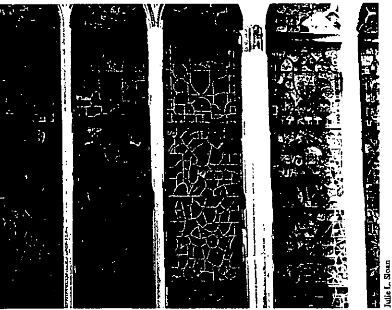
Figure 6: An example of fully leaded protective glazing. The protective glazing is almost indistinguishable from the stained glass behind it.
